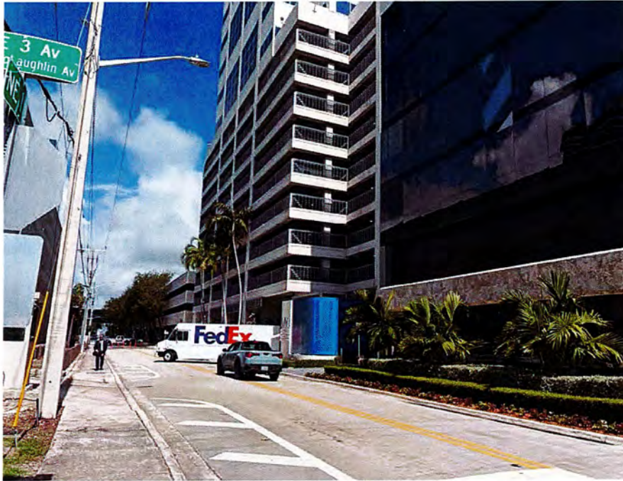
VIEW WEST AT NE 1 ST STREET. PUBLIC PARKING GARAGE ON RIGHT IN BACKGROUND.
