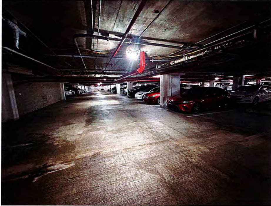
BASEMENT PARKING GARAGE
