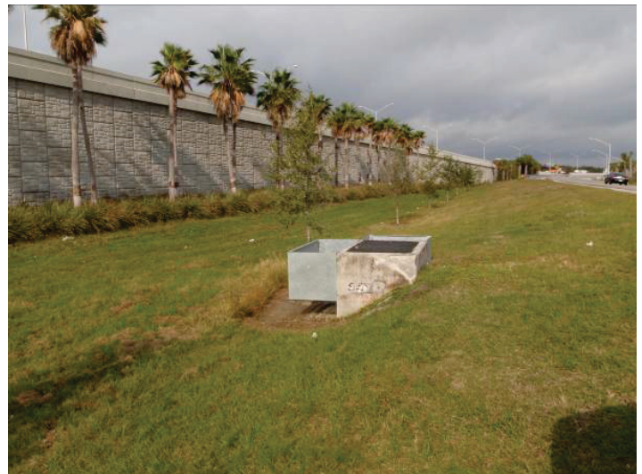
Drainage swale and control structure
