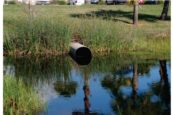
Outfall to stormwater pond
