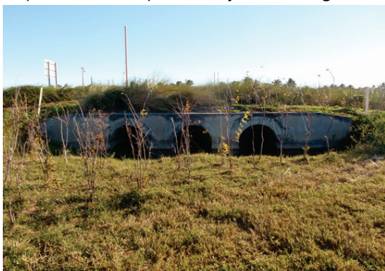
Outfalls to swale along interstate
