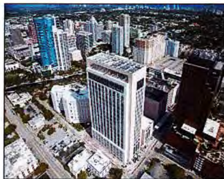
Broward County Courthouse
