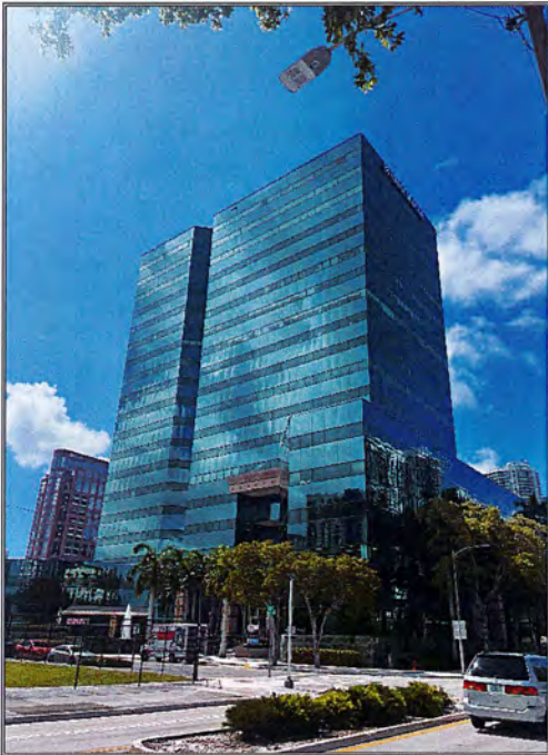
LOOKING SOUTHEAST AT SUBJECT OFFICE BUILDING (FROM N.E. 1 ST STREET)
