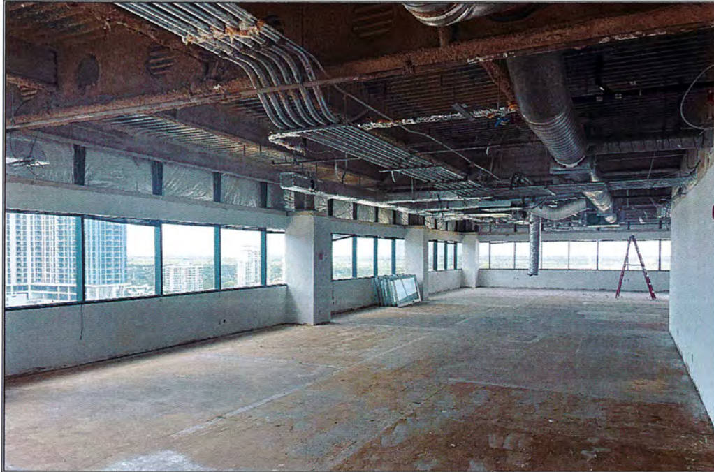
OFFICE INTERIOR VIEW – SUITE 1600 (VACANT SHELL OFFICE)
