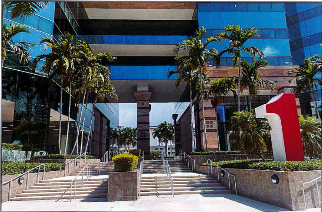
SOUTH SIDE OF BUILDING FACING NORTH
