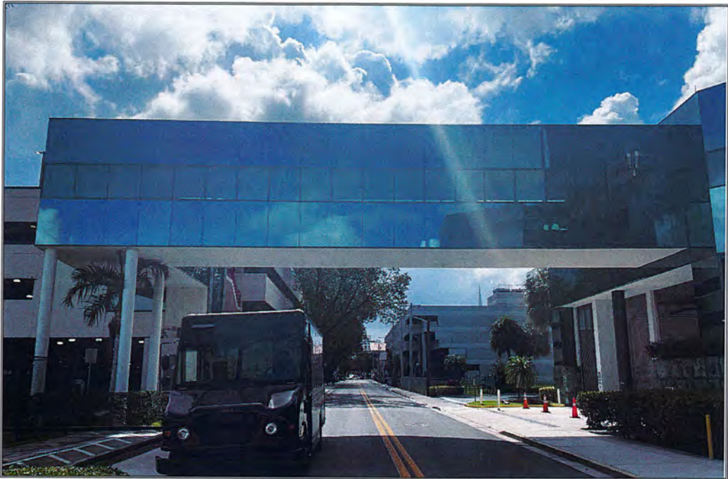
NORTH SIDE OF BUILDING FACING EAST TOWARDS GARAGE PEDESTRIAN BRIDGE
