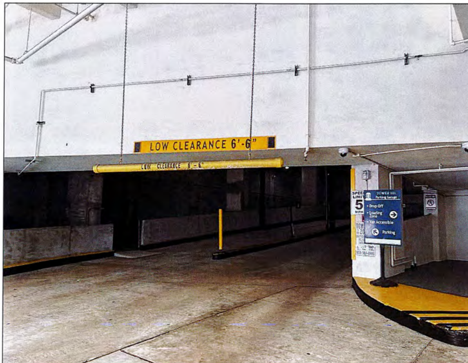
VIEW OF PARKING GARAGE ENTRANCE
