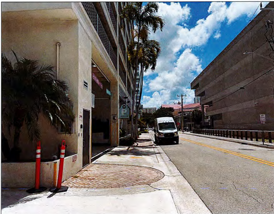
VIEW OF GARAGE ENTRANCE FACING EAST ALONG NE 1 ST STREET
