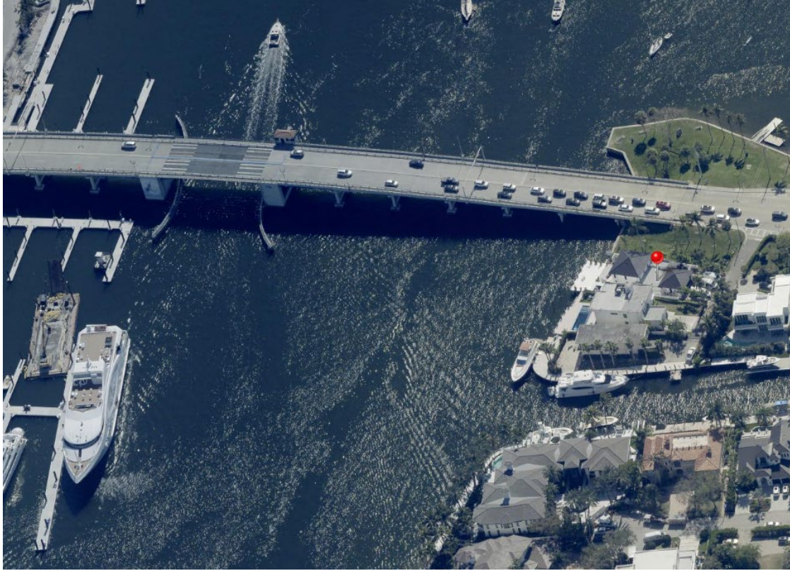
3. North portion of property, facing south.
