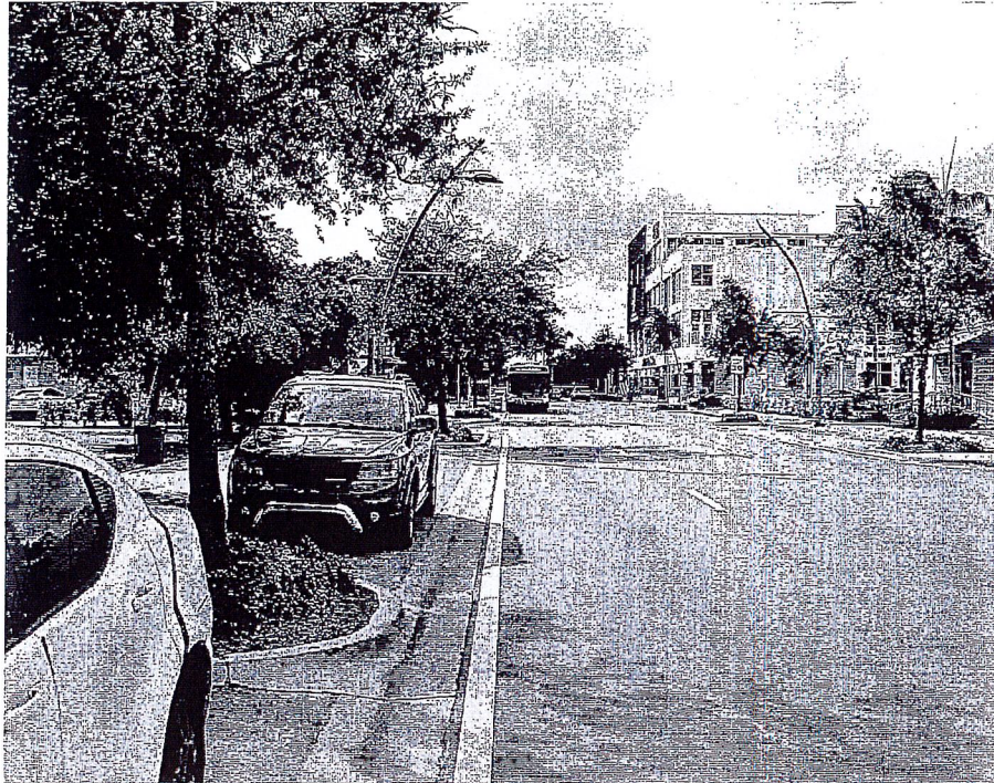
NW 6 STREET, LOOKING WEST
