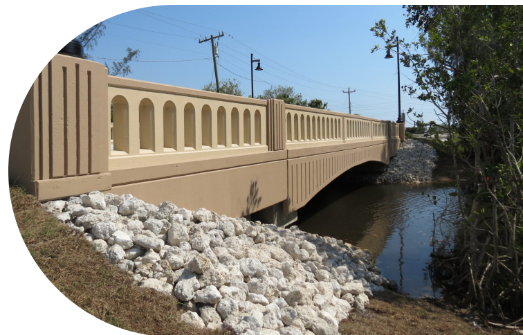
Melbourne Street Bridge - Florida
