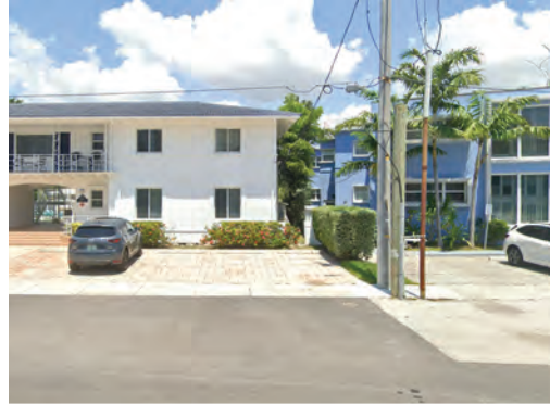
2- SOUTH ON BAYSHORE DR. FACING NORTH
