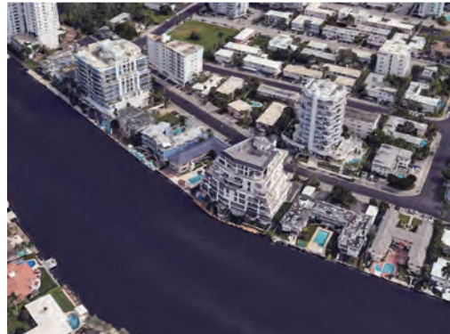
6 - SOUTHWEST CORNER SHOWING NEIGHBORING PROPERTIES
