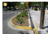
3 Curb Extension with Chase Cover. Source: NACTO
