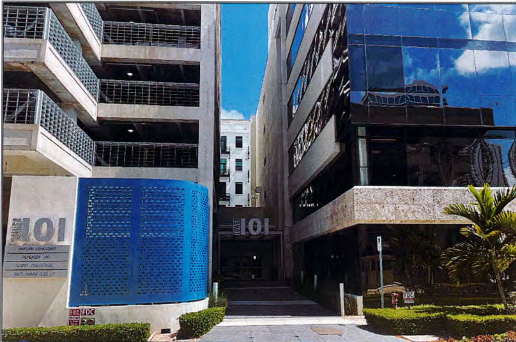
SOUTH SIDE OF BUILDING FACING NORTH
