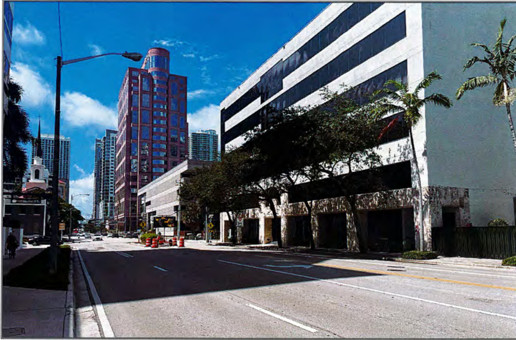
WEST SIDE OF BUILDING FACING SOUTH TOWARDS BROWARD BOULEVARD
