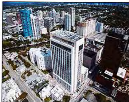
Broward County Courthouse
