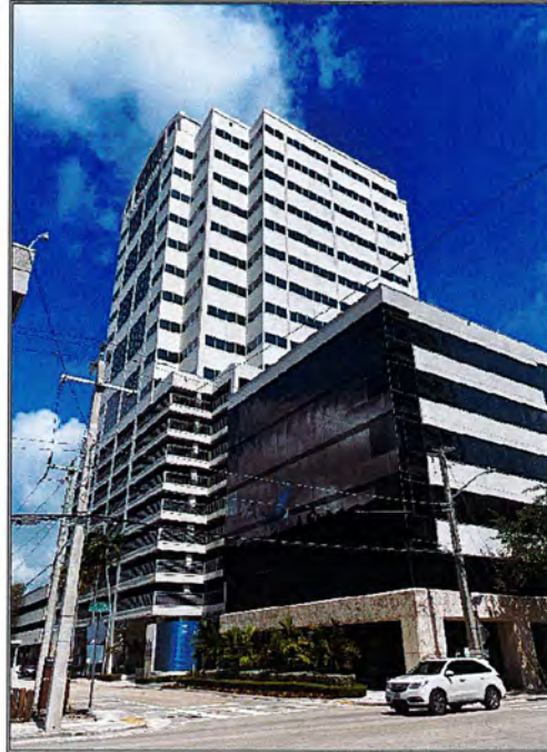
LOOKING NORTHWEST AT SUBJECT OFFICE BUILDING (FROM 3 rd AVENUE)
