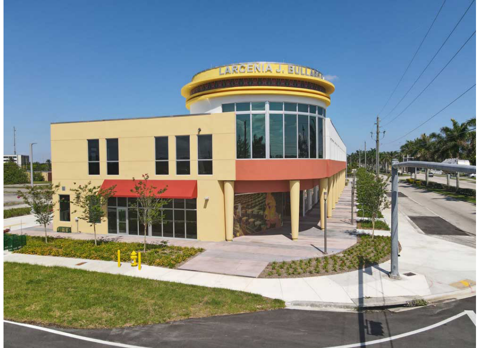
Laura Llerena & Associates was a subconsultant on the design of the Larcenia J. Bullard Building for Miami-Dade County. New 15,000 sf two-story building with retail space, a take-out restaurant and a gallery space on the 1st floor to showcase the history and art of the local Richmond Heights area. The 2nd floor has a community multipurpose room and office space. The project scope includes the design of the entire site with 48 parking spaces. The building achieved LEED Silver Certification.
