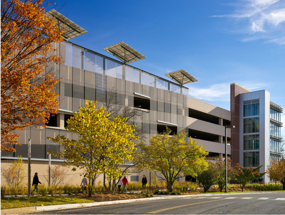
The Universities at Shady Grove P2 in Rockville, Maryland received Parksmart Bronze Certification. This was achieved by incorporating multiple pay stations, tire inflation station, electrical vehicle charging stations, natural ventilation, high-efficiency lighting, and on-site photovoltaic array on roof.
