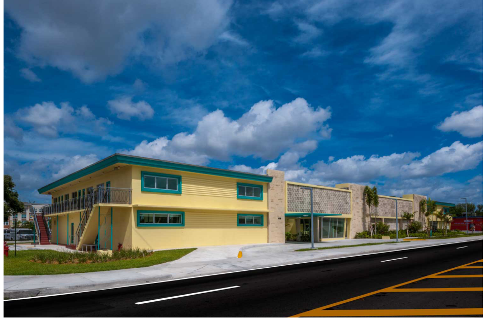
In 2016, Gurrimatute completed the restoration and adaptive reuse of the Historic Hampton House with O'Donnell & Naccarato (formerly Douglas Wood & Associates) and Laura Llerena & Associates. This historic preservation project received numerous awards including from AIA Miami, AIA Florida, and Dade Heritage Trust.
