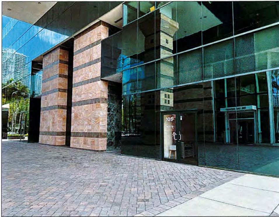
VIEW OF GROUND FLOOR RESTAURANT
