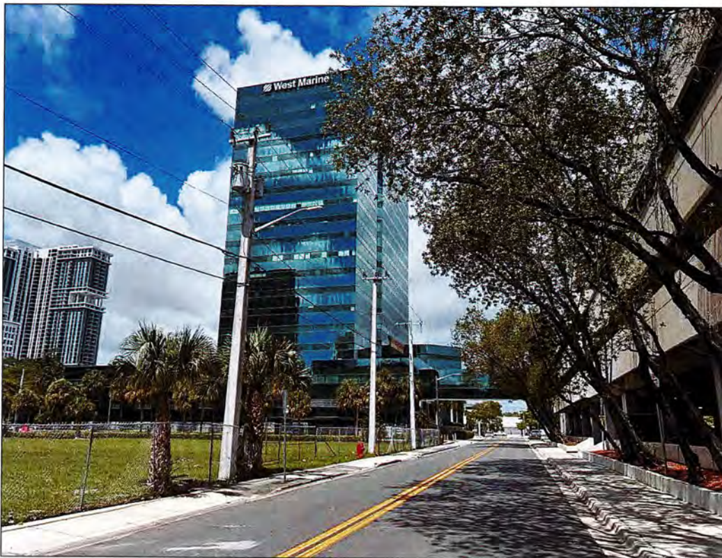
1 EAST BROWARD AND PEDESTRIAN BRIDGE TO PARKING GARAGE
