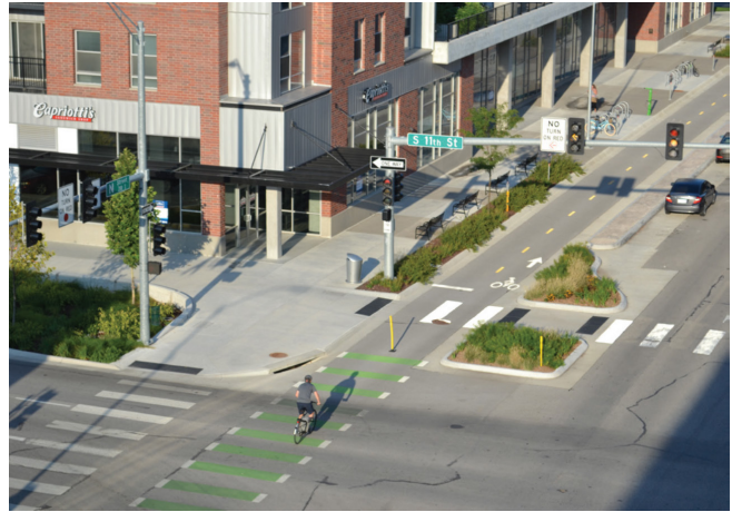
Alta specializes in finding the best design solutions to balance budget and function, and can seamlessly marry streetscapes and green street treatments with traffic analysis, signal design, and roadway geometrics.
