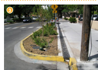
3 Curb Extension with Chase Cover. Source: NACTO
