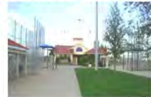
Spanish River Athletic Facility
