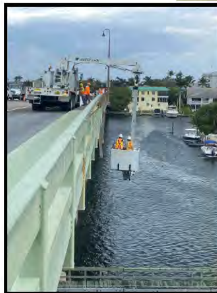
Linton Boulevard Bascule Bridge
