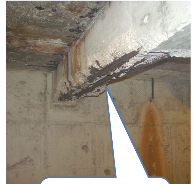
Filter structure exposed rebar repaired in 2012
