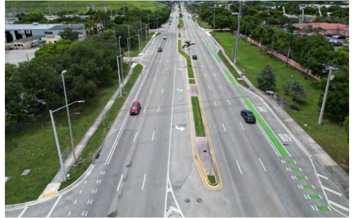
MARLIN FDOT D4 Powerline Road Improvement Project
