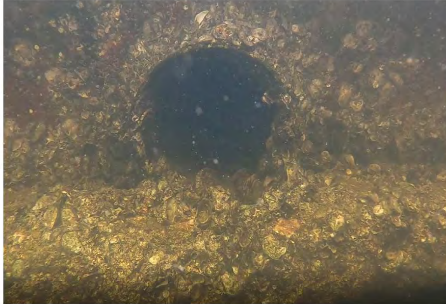
Photo 7 – Photo of survey area. Note outfall and oysters on sea wall.
