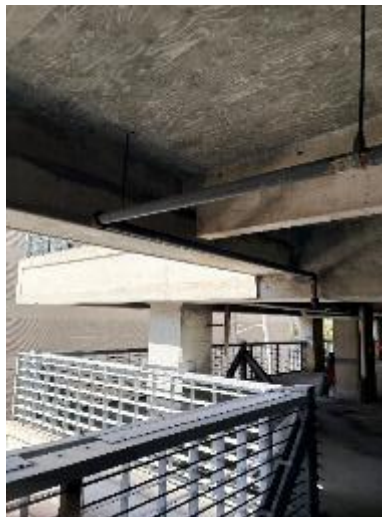
Figure 2B.2.2 Garage railings
