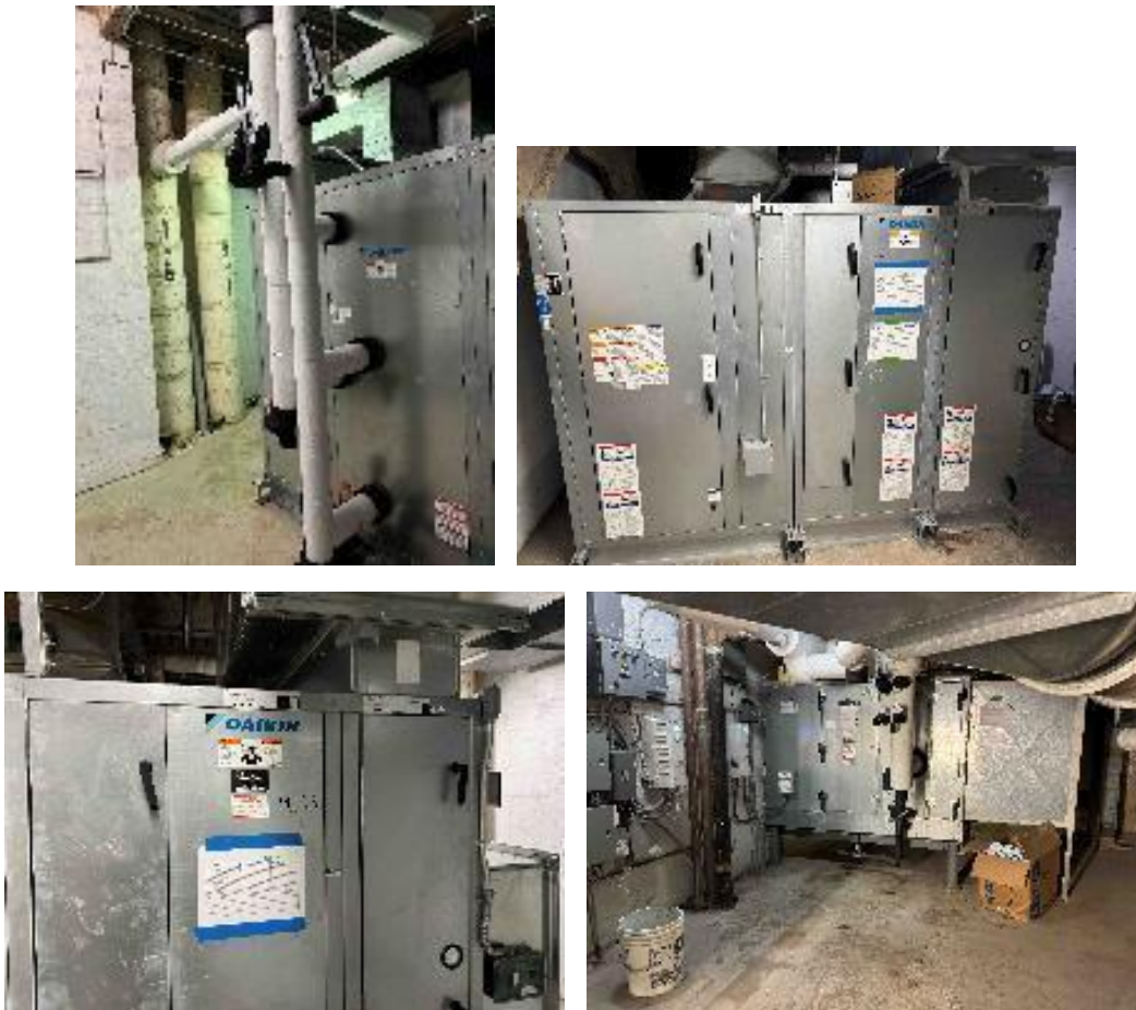
Figure 2A.4.3 AHUs in good condition
