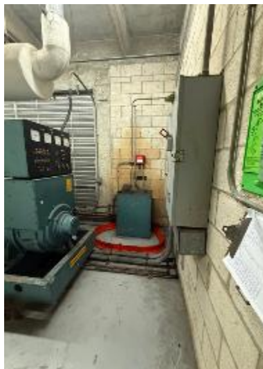
Figure 2B.6.15 Emergency generator working clearance (Center)
