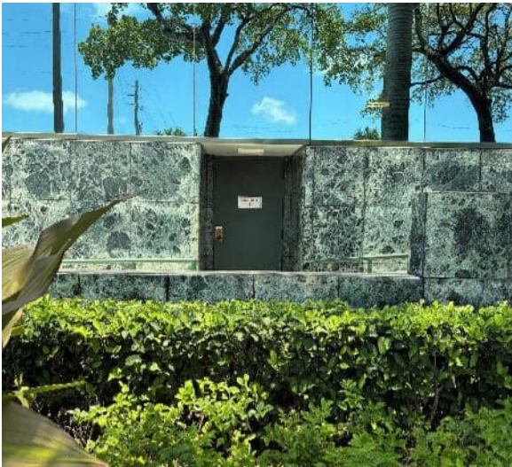
West side of building. Egress stair. Approx 2' above grade. Stairwell will take on water.
