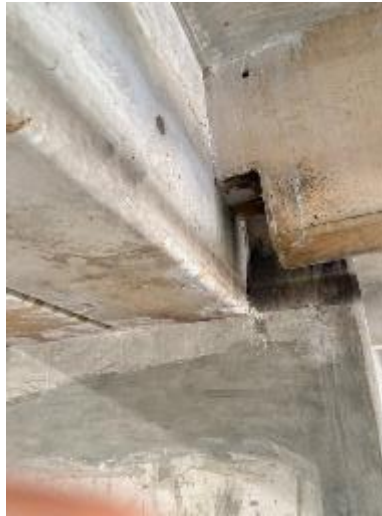
Figure 2B.2.3 Precast joists
