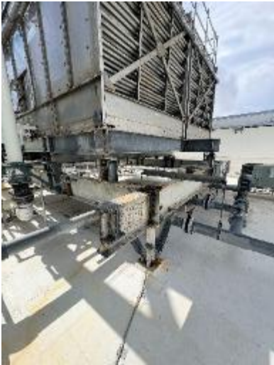
Figure 2A.2.4 Cooling tower framing
