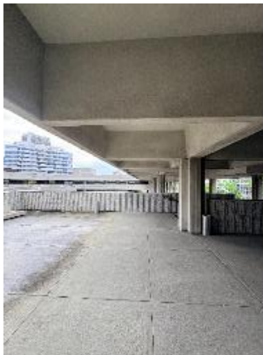
Figure 2C.2.2 Typical exterior precast soffits
