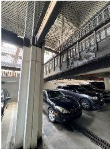
Figure 2C.2.1 Bridge surface appearance
