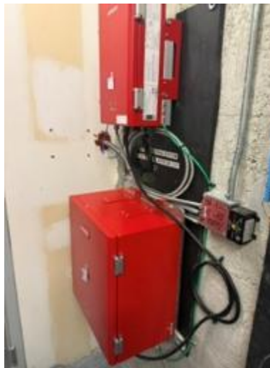
Figure 2B.5.2 Bi-directional amplifier
