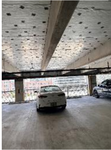
Figure 2B.2.1 Under slab insulation
