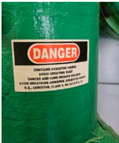
Figure 2C.4.3 Sample label on insulation
