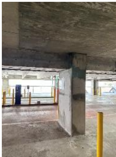
Figure 2B.2.4 Garage structure
