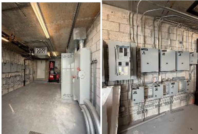
Figure 2B.6.21 Rooftop electrical equipment
