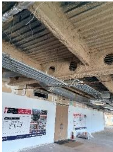
Figure 2A.2.2 Mechanical penetrations at girders
