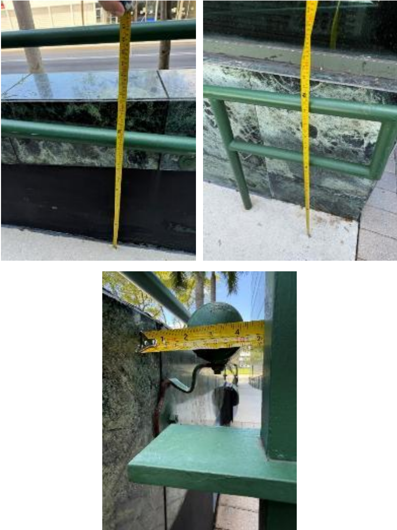
Figure 2A.3.9 Exterior Ramp Railing
