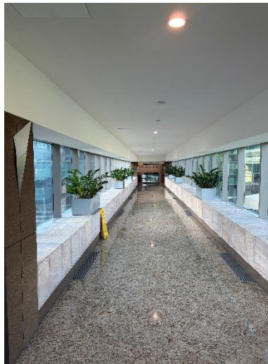
Figure 2A.3.20 Pedestrian bridge
