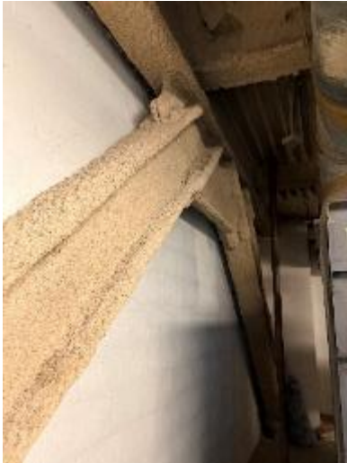
Figure 2A.2.3 Typical main wind-force resisting system
