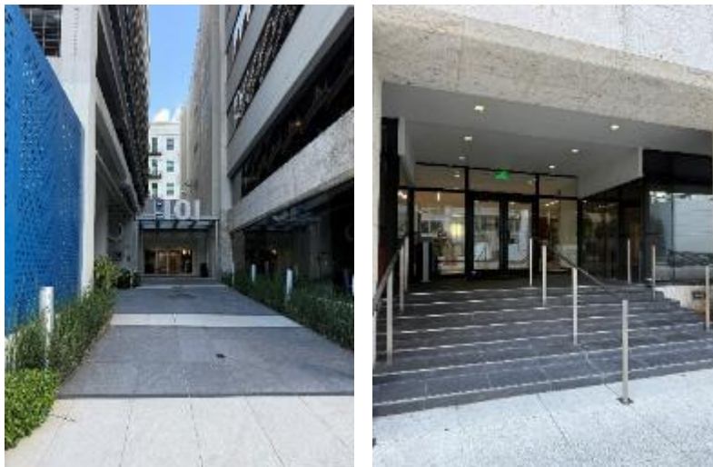
Figure 2B.3.7 Exterior access
