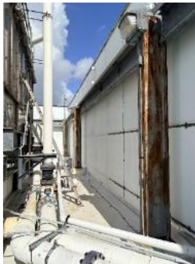
Figure 2A.2.6 Rooftop screen wall framing
