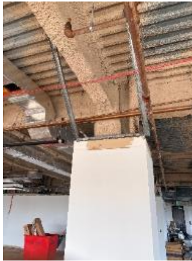
Figure 2A.2.1 Underside of floor framing
