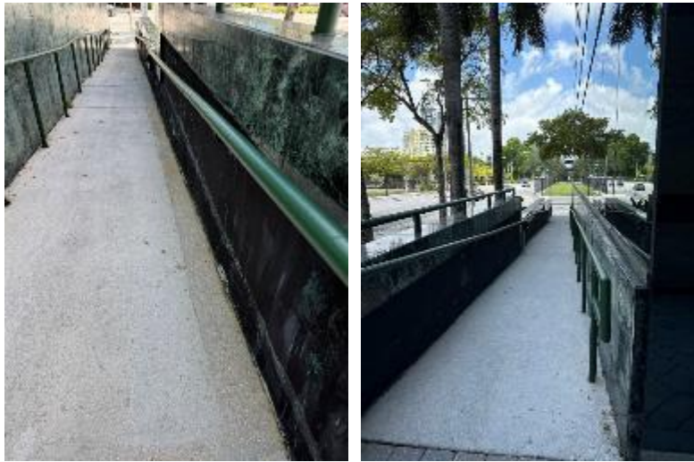
Figure 2A.3.7 Exterior Ramp
