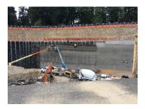
This project calls for the construction of a new 17.4 million gallon, seismically reinforced below ground reservoir, within the footprint of the existing reservoir 3 (upper) with a reflection pool/water feature on top. Designed to retain the historic look and feel of the original reservoir, it has been engineered to withstand ongoing landside encroachment and potentially catastrophic effects of a major earthquake.
