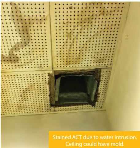
Roof leaks and ceiling stains yet to be replaced.
