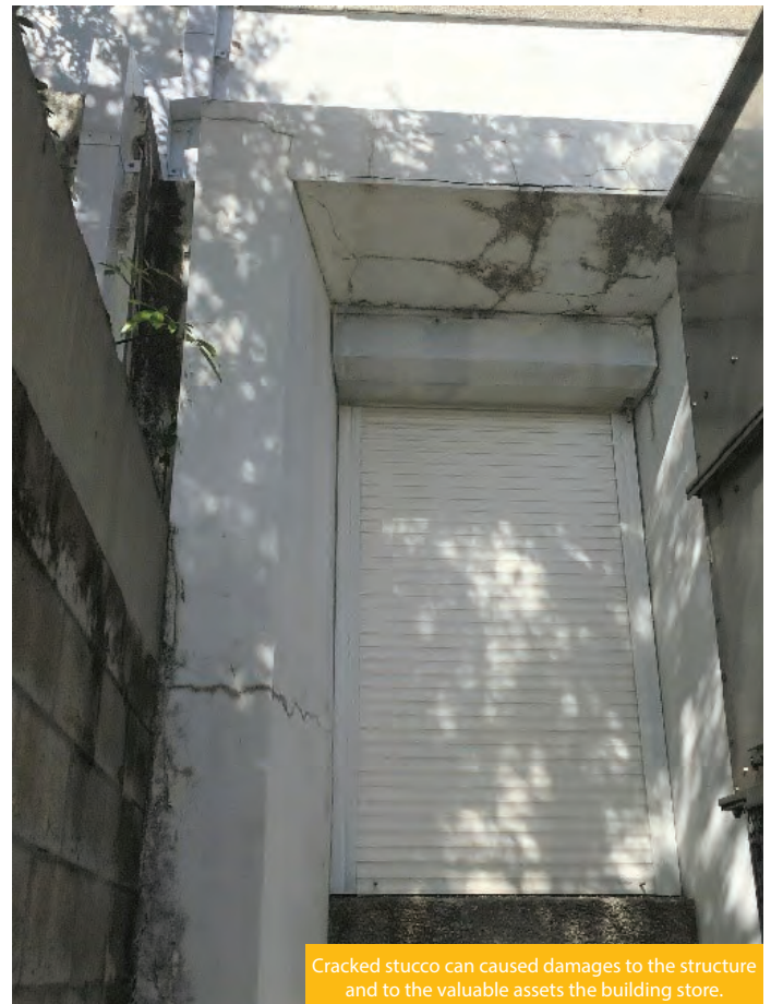
Front Facade. Cracked stucco and deterioration of the building causing damages and an unattractive appearance.
