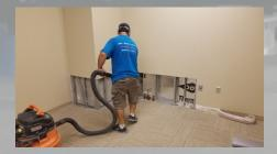
United Restoration maintaining a clean workspace after executing an emergency dry-out and removing water damaged drywall.
