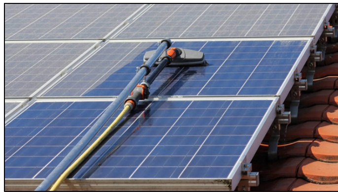
Figure 5: Basic maintenance routine of an array (source: energymatters.com). Removing dust improves efficiency by 1%.
