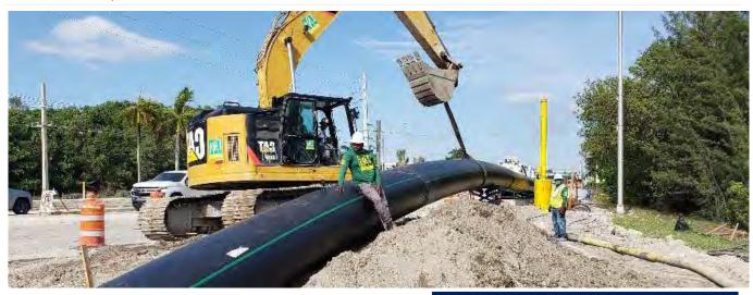
This project consisted of construction of a 48-inch force main by directional drill, open cut, and slip-lining methods. Existing linestop and 24-inch bypass was installed as part of the scope of work of RPQ PO231 by DMSI. The work zone was restored by completing pavement resurfacing and bringing pavement marketing and signalization up to specifications.
