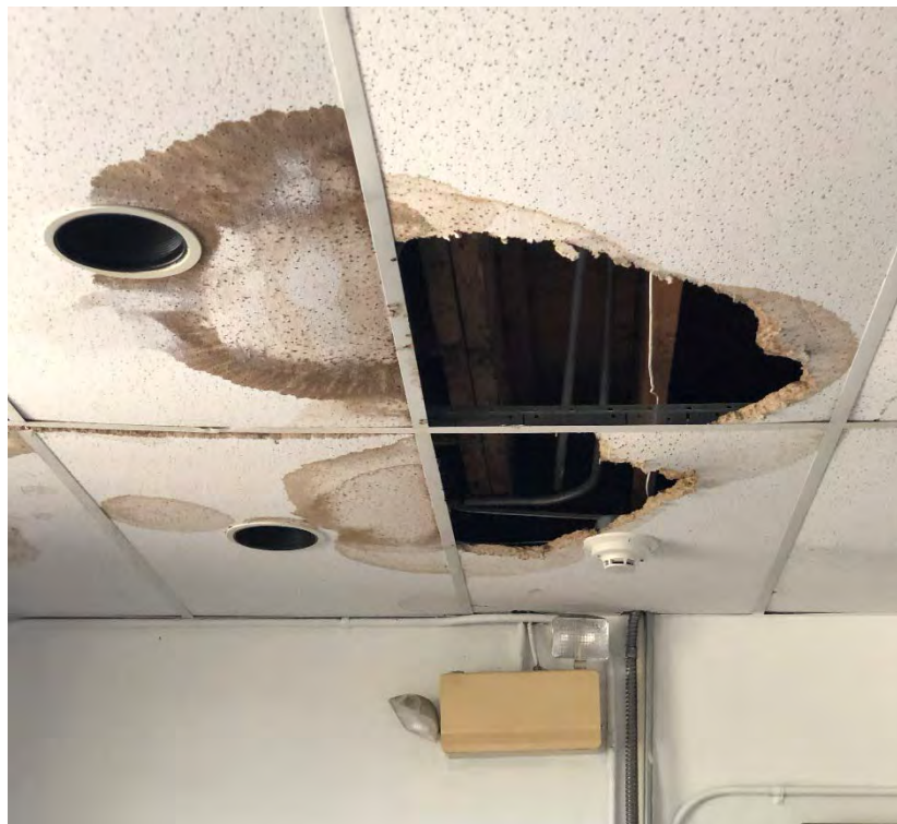
EVIDENCE OF WATER LEAK IN CEILING
