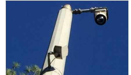
CCTV CAMERA AND TRAFFIC SENSOR (MDVS)
