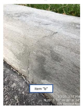
I. Trip hazard between Type D Curb and Concrete Sidewalk STA 30+71.
