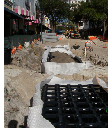
SUSPENDED PAVEMENT SYSTEM INSTALLATION, CLEMATIS ST
