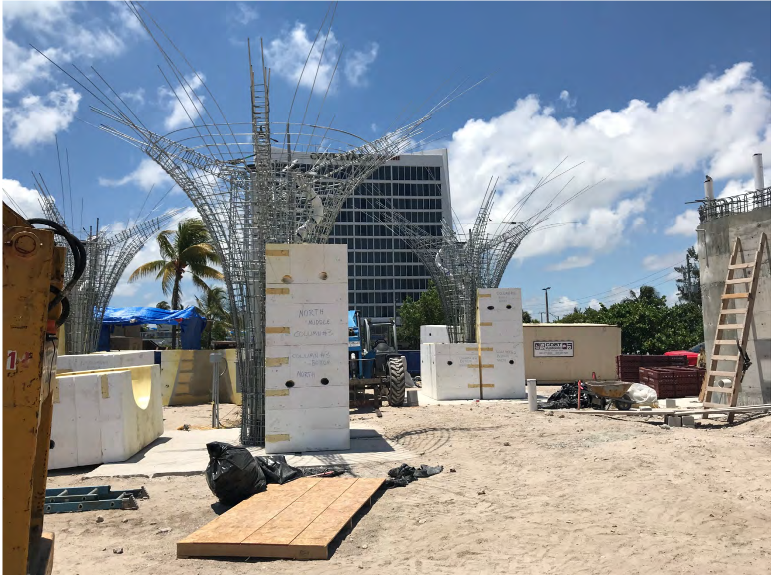
OCEANSIDE PARK PROGRESS PHOTO TAKEN ON 5-23-2019 (SHADE CANOPY REBAR AND FORMWORK - FACING SOUTH)
