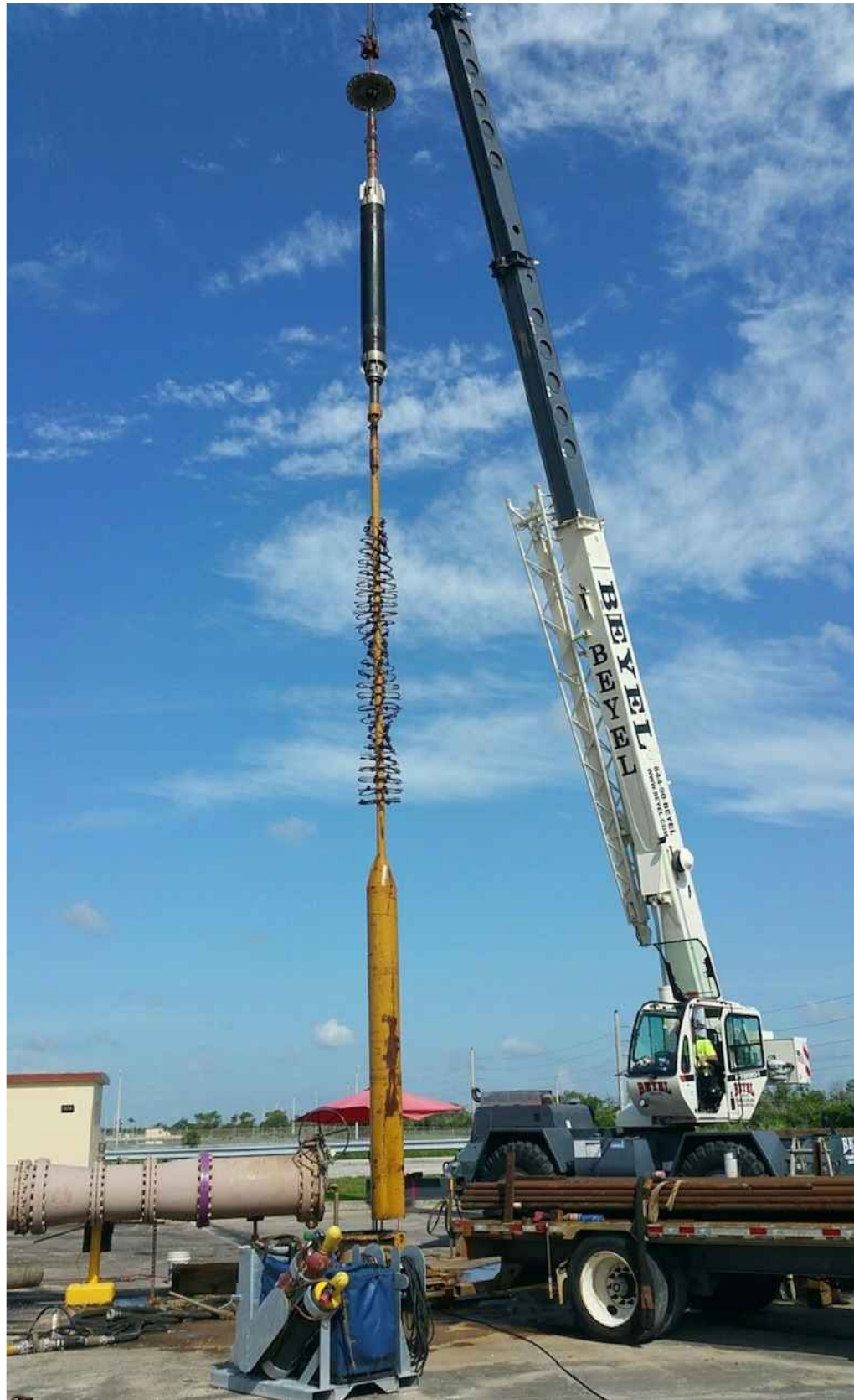
Figure No. 13 City of Fort Lauderdale G.T. Lohmeyer Injection Facility Image of Typical Casing Brushing Tool Configuration
