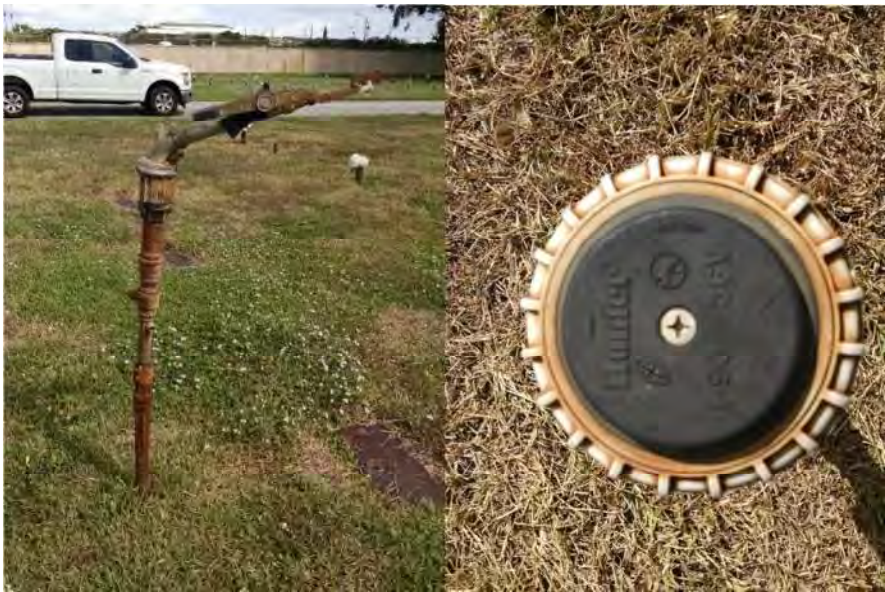
Figure 20 - Above grade impact rotor and modern rotor found on-site.
