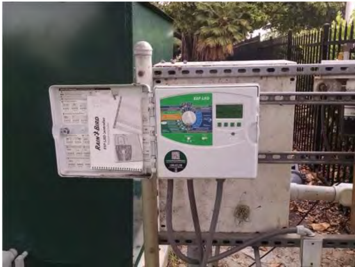
Figure 14 - Rain Bird ESP-LXD 2-wire controller at South pump station.
