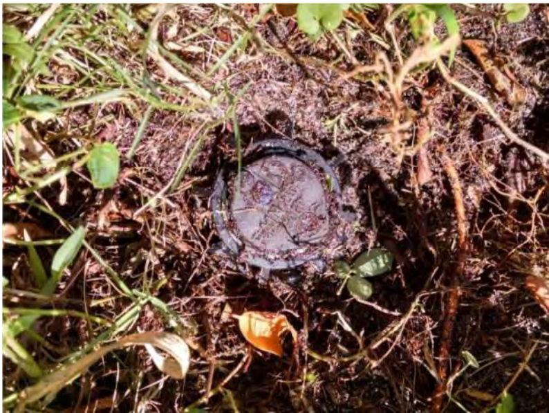
Figure 4 - Rain Bird 5000 head in ground.
