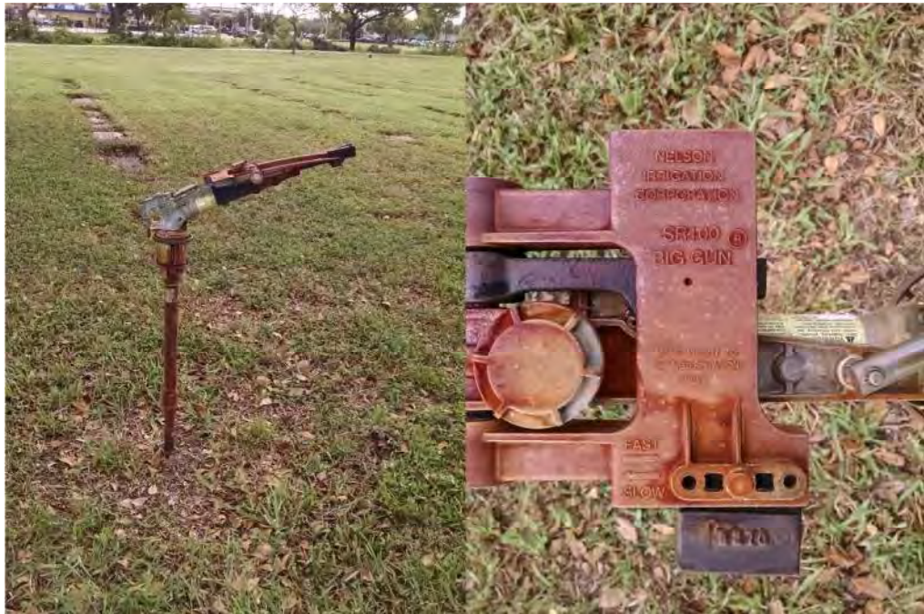
Figure 11 – Nelson SR 100 impact rotors found in East half of park.
