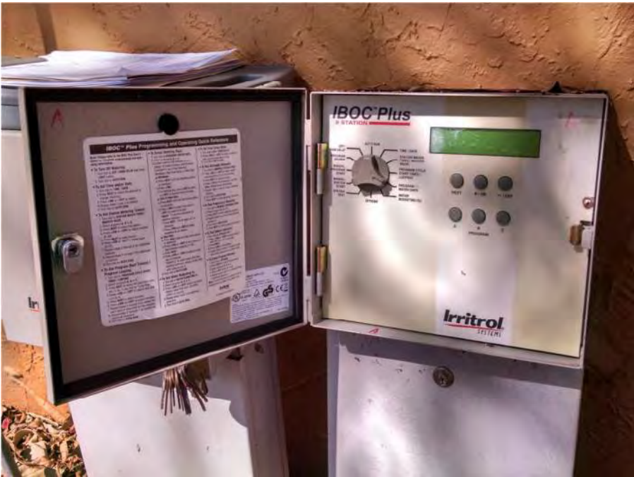
Figure 28 - One of two controllers found on-site. Neither controller currently was powered.
