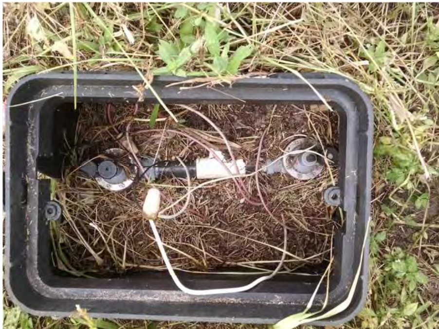
Figure 18 - Typical low flow valve on-site.
