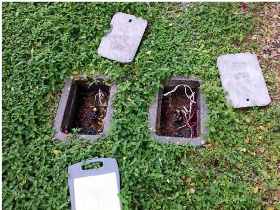
Figure 26 - Typical valves found on-site (concrete valve boxes).
