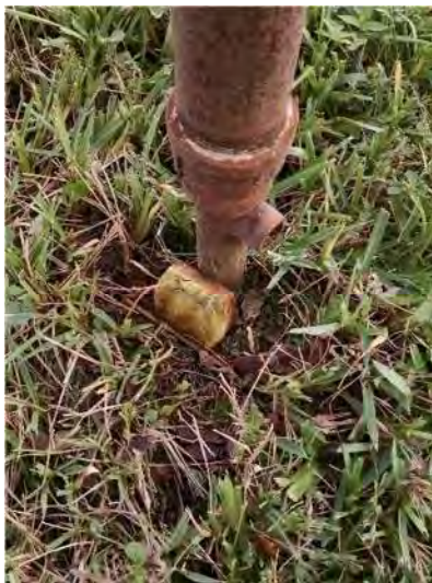
Figure 9 - Quick coupler for impact rotor use.
