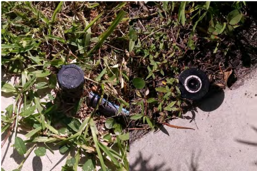
Figure 21 - Bubbler and spray heads found on-site.
