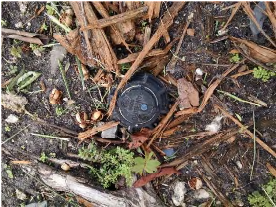
Figure 12 - Rain Bird 5000 head found in West half of park.
