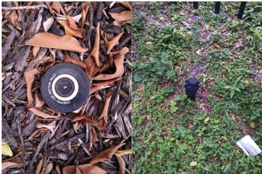
Figure 27 - Spray and rotor heads found on-site.
