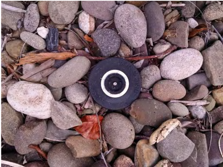
Figure 13 - Rain Bird 1800 head found in West half of park.
