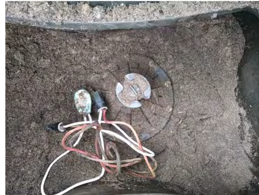
Figure 10 - Typical Rain Bird PGA RCV, note silt/sediment depth.
