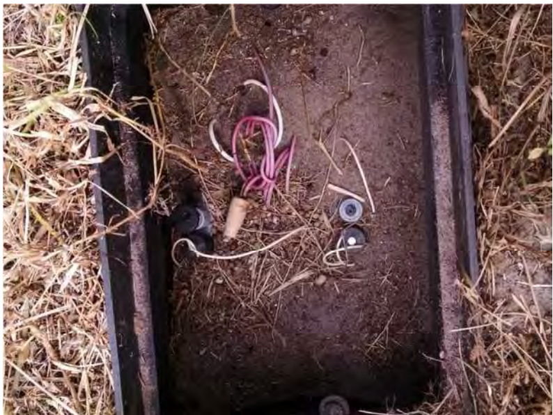
Figure 19 - Typical valve found on-site. Note silt/sedimentation.
