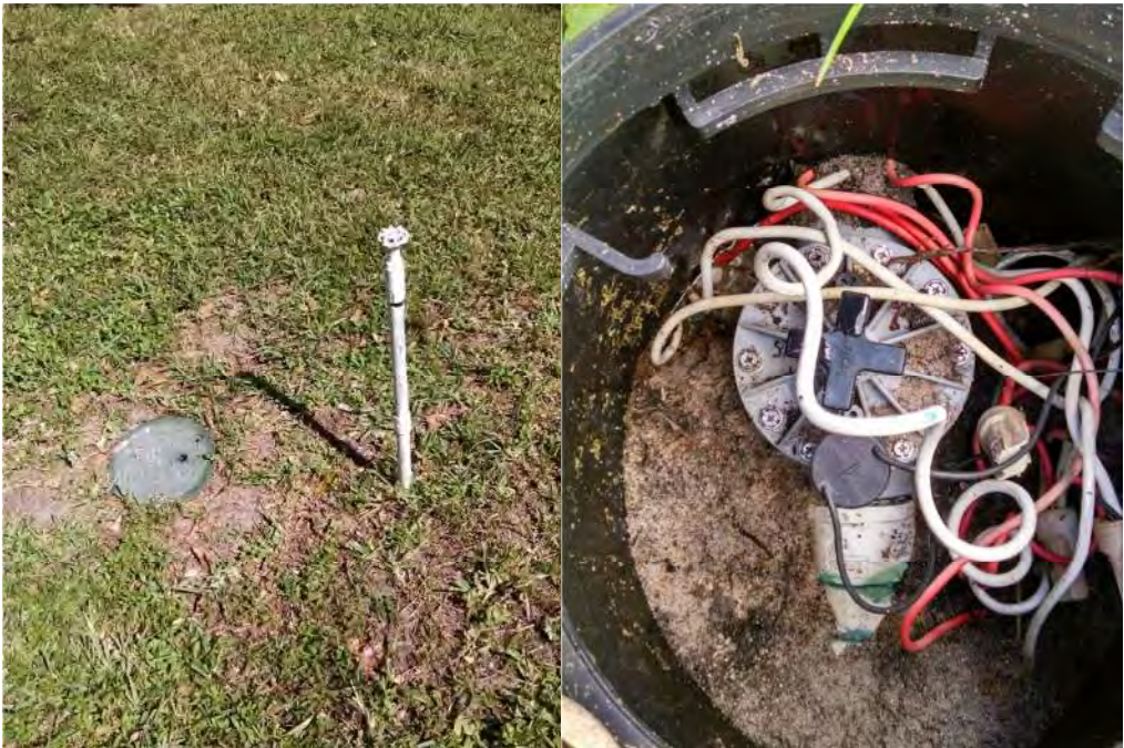
Figure 3 - Valve and hose bib (typ.) on left. Valve with associated wiring on right.
