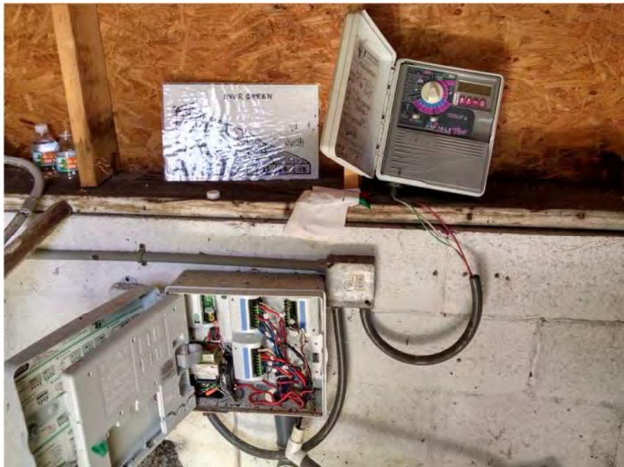
Figure 5 - Evergreen Cemetery controllers. ESP-LXME in lower left (in-use) and ESP LX-16 Plus in upper right (currently unused).
