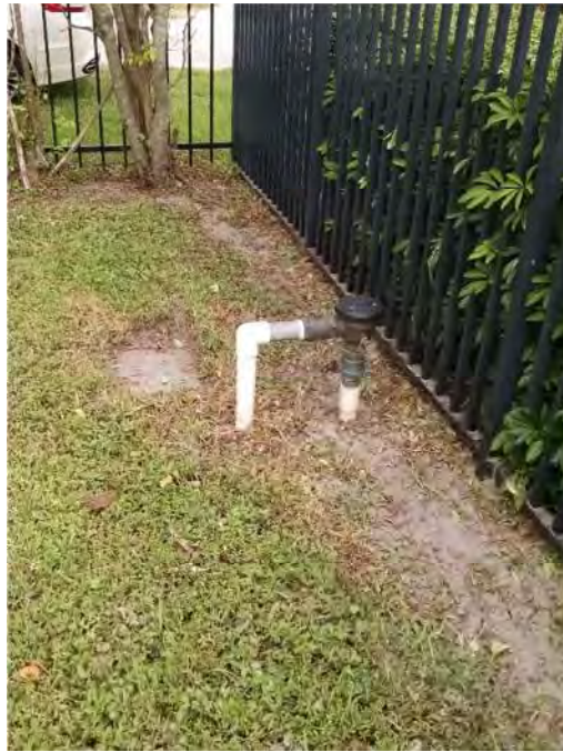
Figure 8 - Typical water meter and backflow device (Northeast entrance POC pictured).
