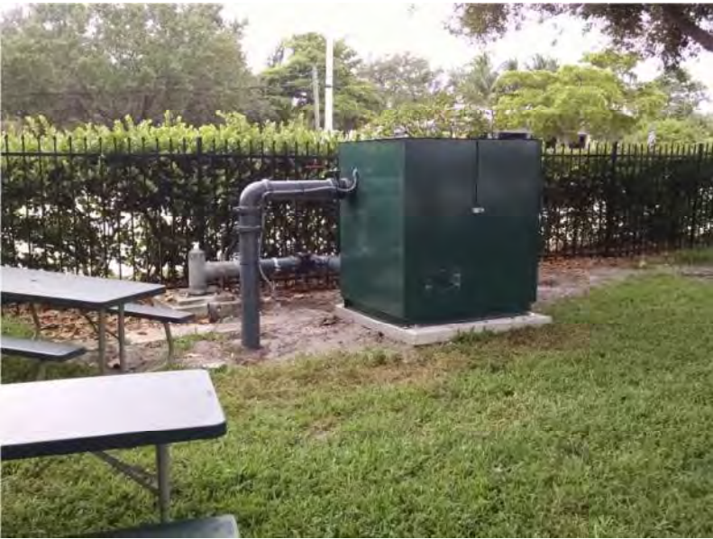
Figure 7 - Typical pump station and well configuration (West well and pump station pictured).
