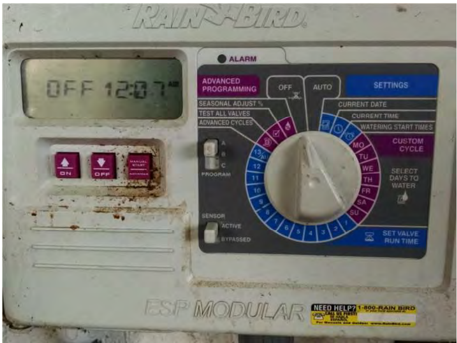
Figure 23 - One of the controllers found in the "off" position.
