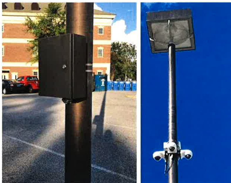
Security cameras and enclosure mounted on a light pole for FoPark's parking occupancy solution
