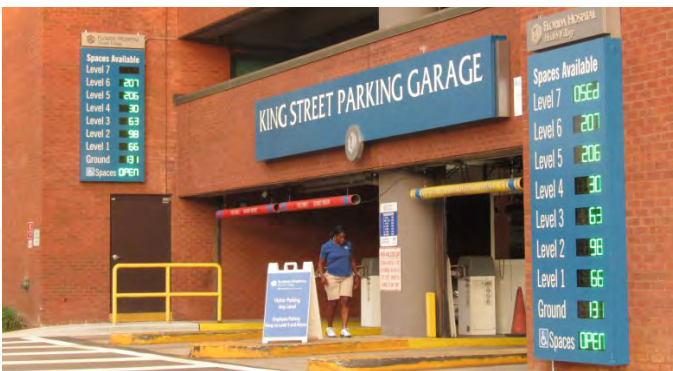
Master panel sign at garage entrance
