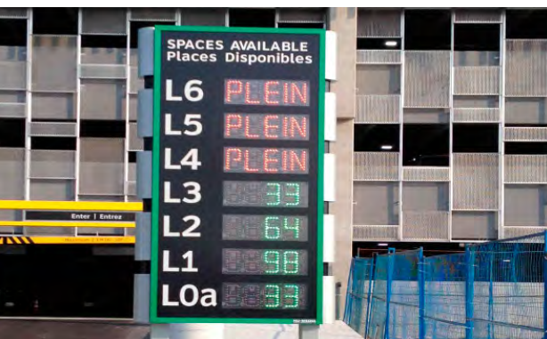
Master panel sign at garage entrance
