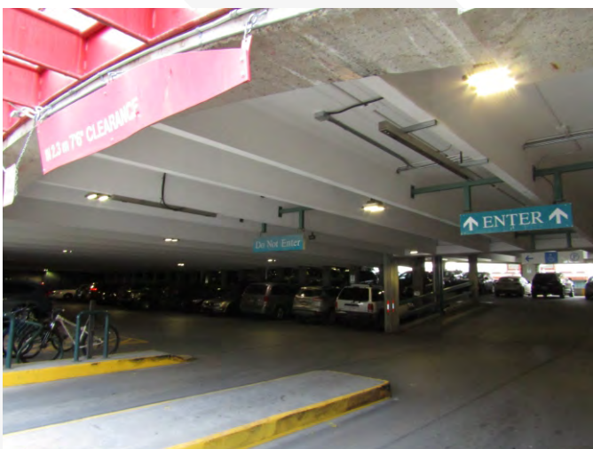
Overhead USDS monitoring parking structure entry/exit
