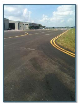
As part of the project, an existing taxiway edge "apron" was removed and three full strength taxiway connectors were constructed to the east shoulder of Taxiway Charlie to eliminate the possibility of aircraft parking within the Taxiway Safety Area. Careful construction phasing was required as access to tenant/fixed base operator ramps and the Customs ramp needed to be maintained during daylight hours.
