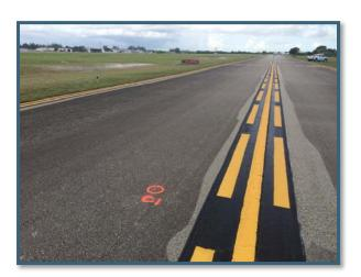
Kimley-Horn used the FAA's Rigid and Flexible Iterative Elastic Layered Design (FAARFIELD) modeling program to determine if the existing pavement sections would be adequate to meet future loading requirements. Based on the analyses, 2 inches of additional asphalt was recommended for the taxiways.
