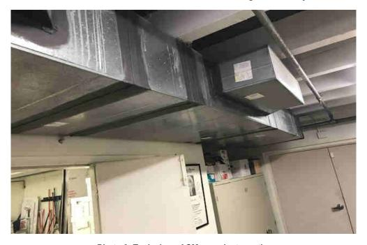
Photo 6: Typical nonACM gray duct mastic.
