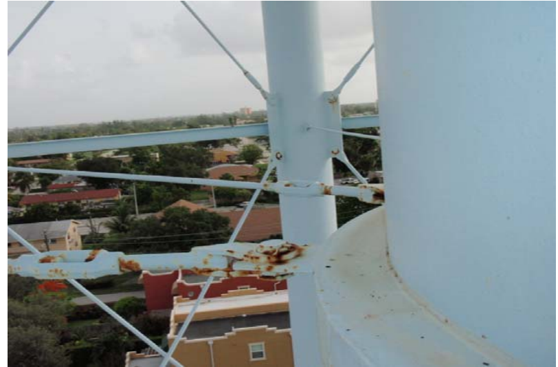
18. Second level riser rods.
