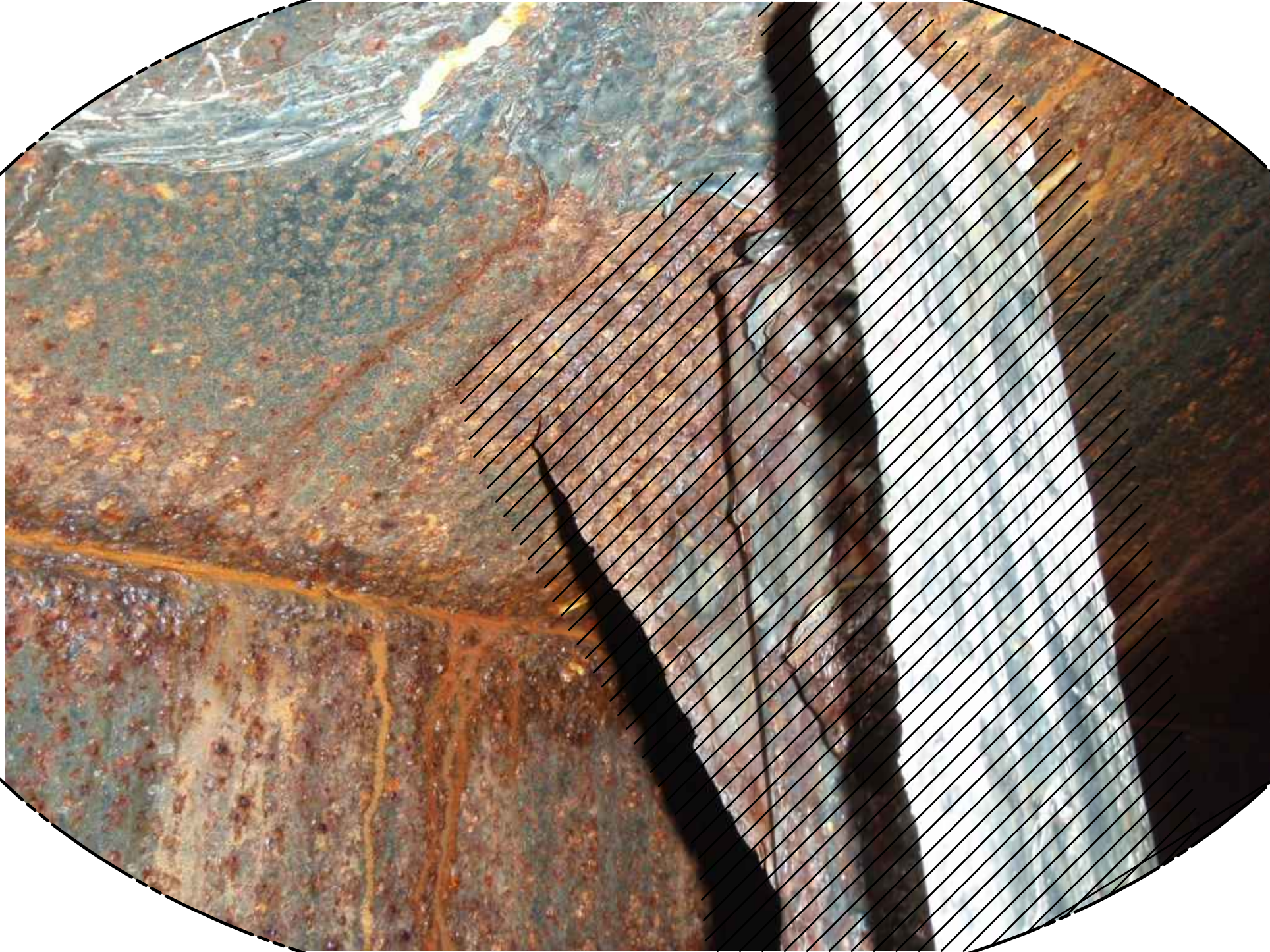
PHOTO 11 – TANK INTERIOR LADDER TOP BRACE NTS
