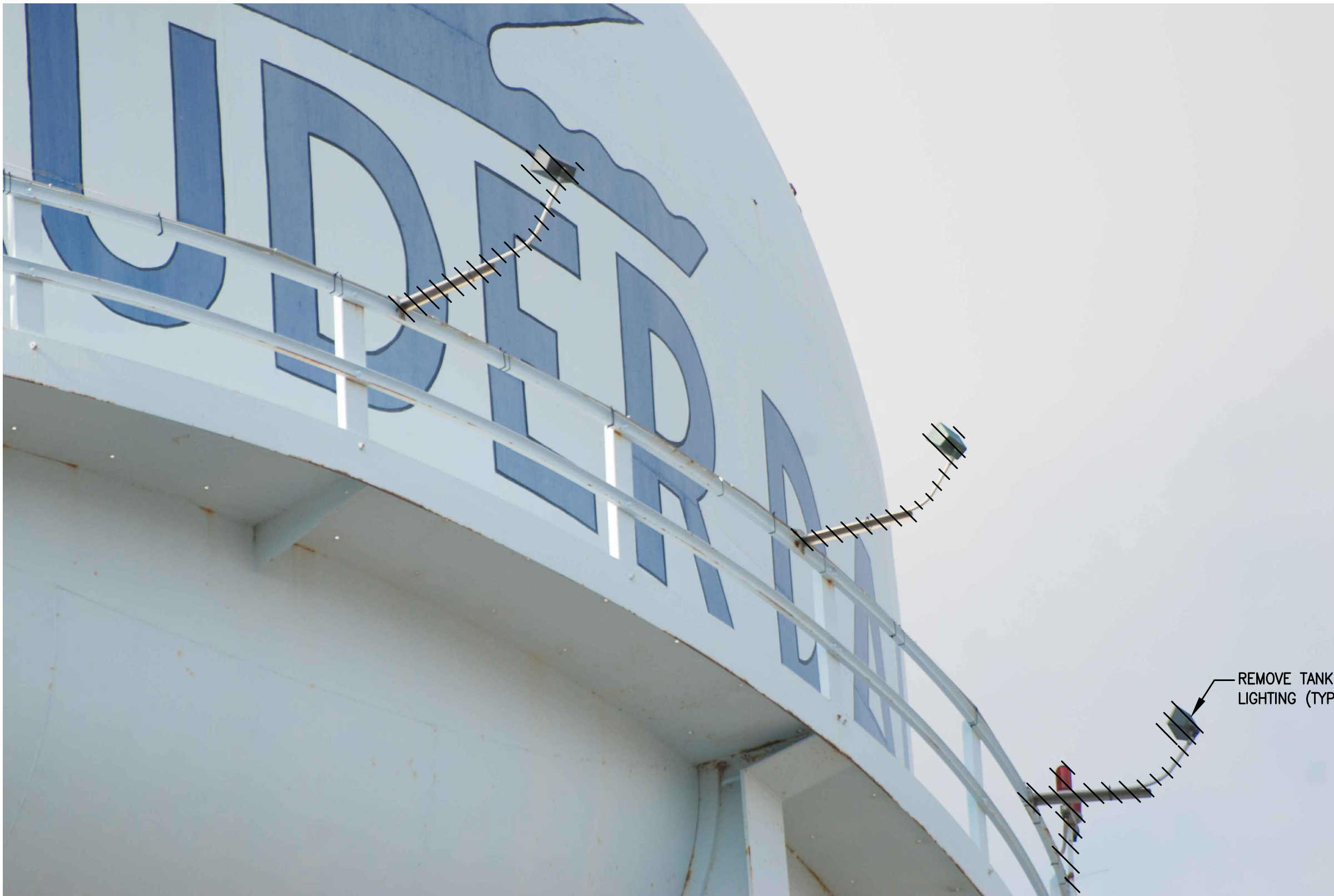
PHOTO 17 – TANK SIGN LIGHTING NTS
