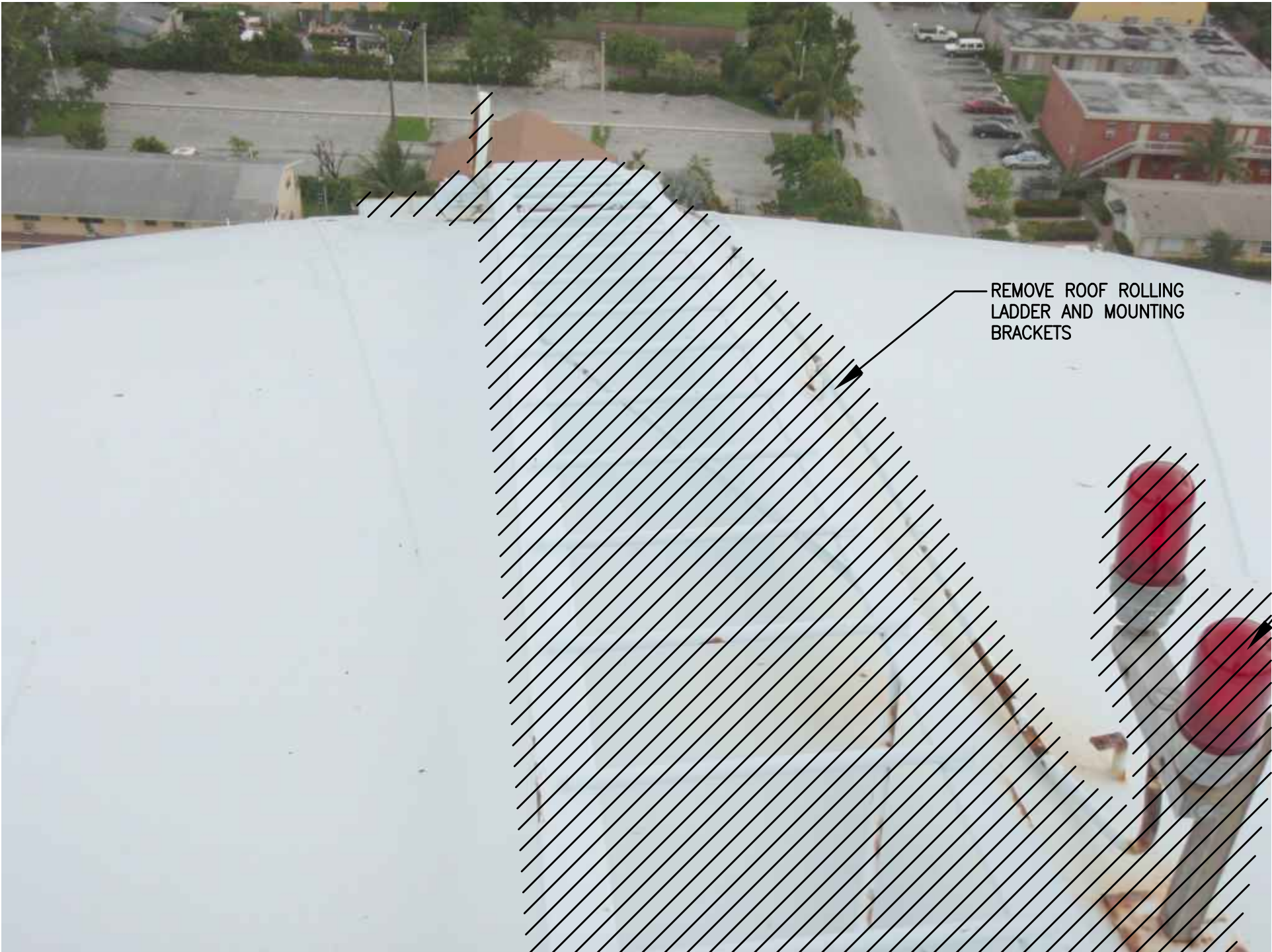
PHOTO 10 – ROOF LADDER AND AIRCRAFT LIGHT NTS
