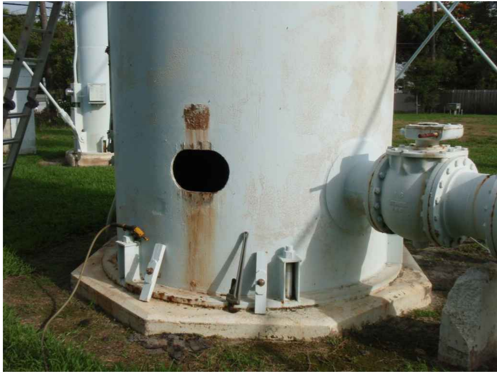
PHOTO 21 – RISER ACCESS OPENING – OPEN HATCH N.T.S.
