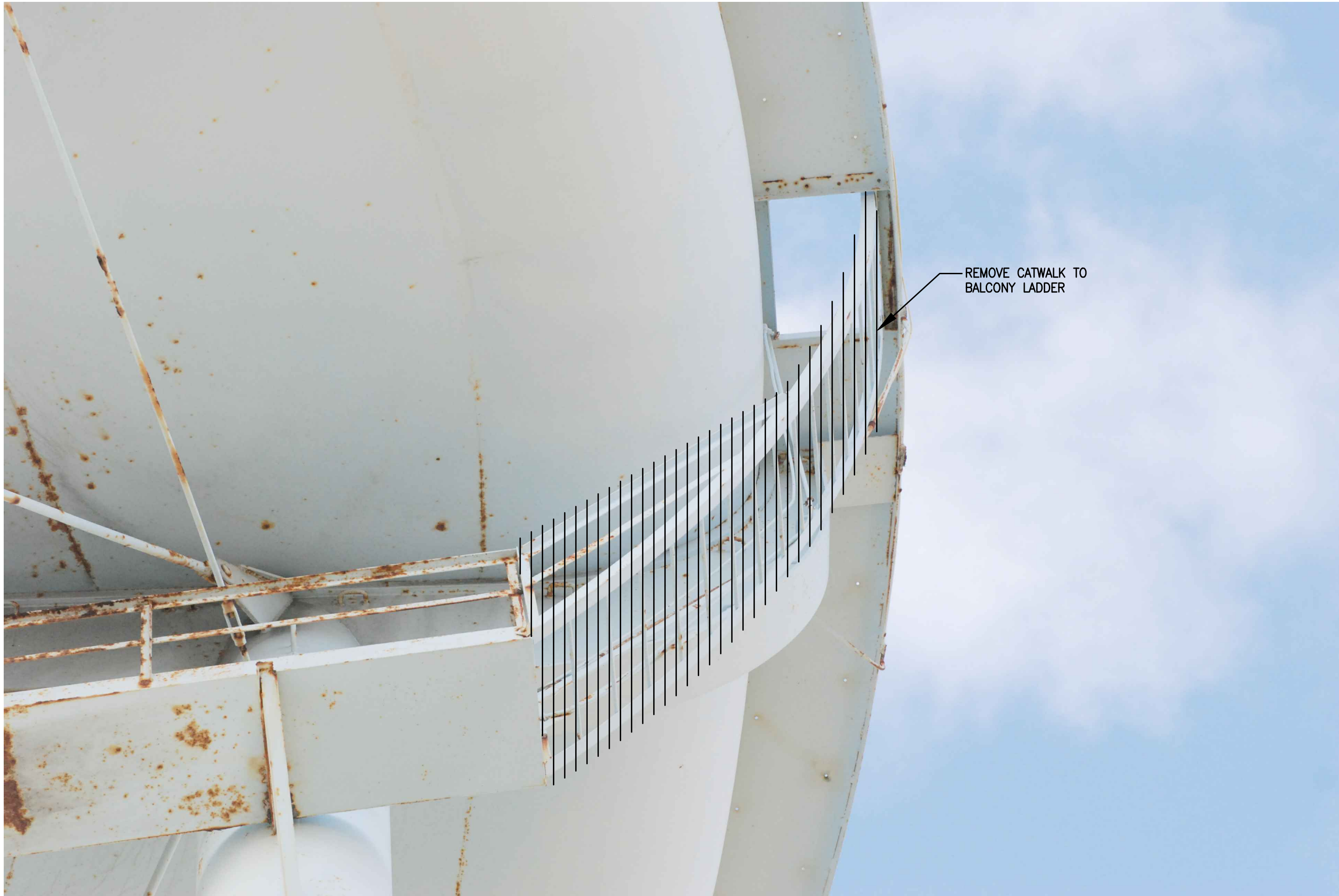
PHOTO 6 – CATWALK TO BALCONY LADDER NTS
