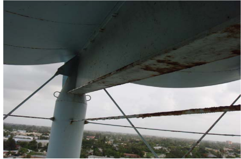
22. Tank support beams.
