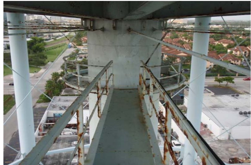
24. Under tank catwalk.
