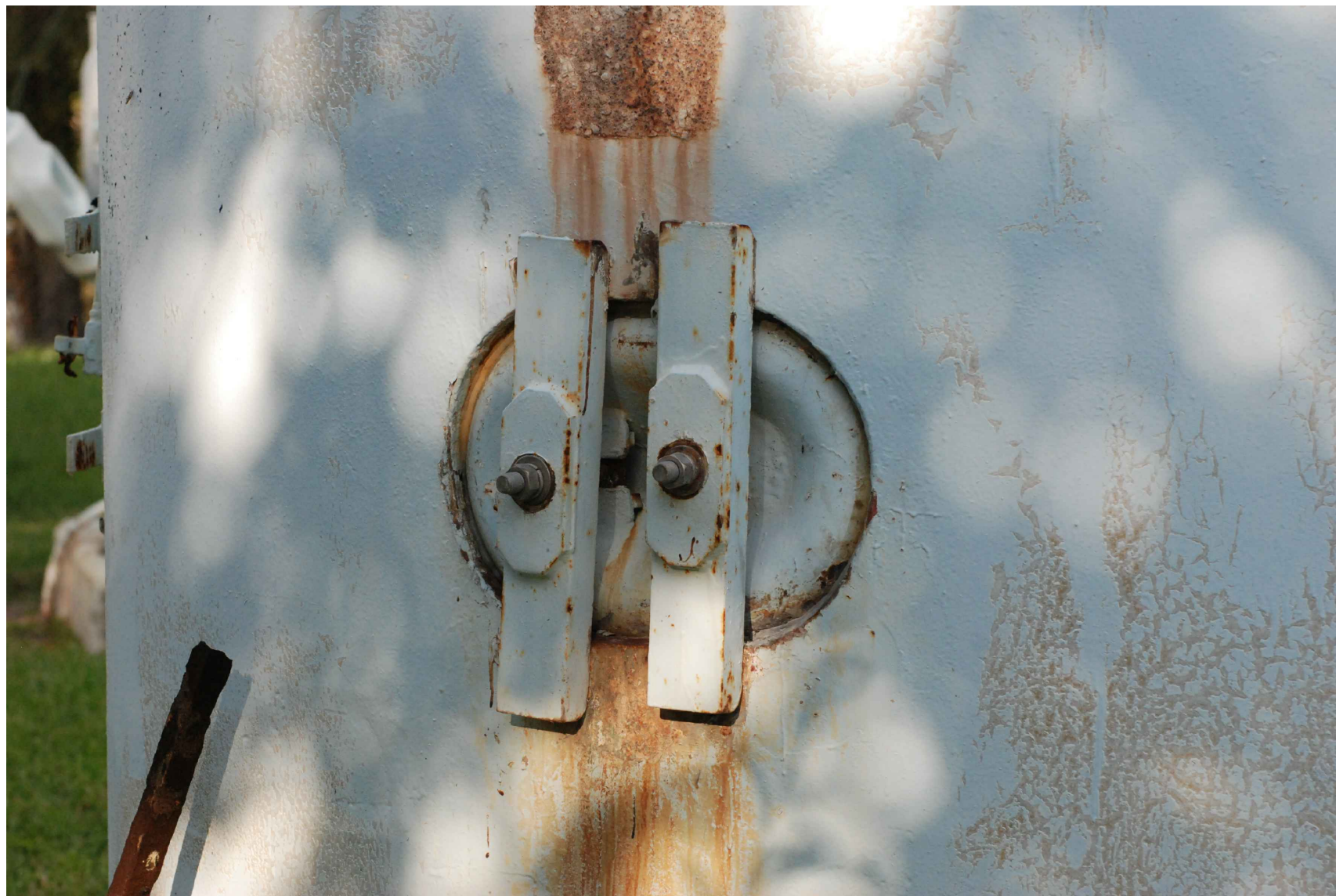
PHOTO 20 – RISER ACCESS OPENING – CLOSED HATCH N.T.S.
