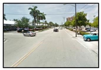
The existing conditions along Cordova Road consist of a 4-lane section within a 70 foot right of way. The roadway has sidewalks on both sides with a landscape buffer in a portion. The existing 46-feet width of paved asphalt is not pedestrian or bicycle friendly. The project length is approximately 970 feet.
