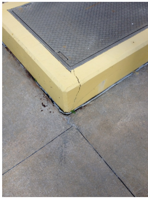
Replace expansion joint around curb (repair of the curb is listed in another category).
