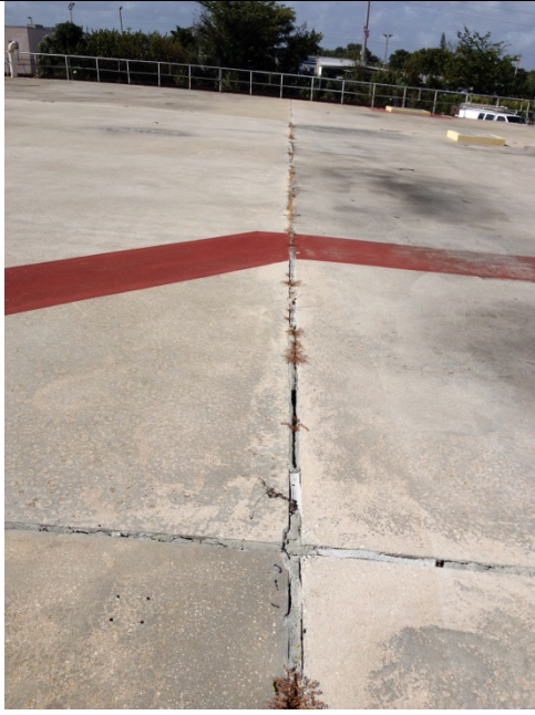
Replace expansion joint
