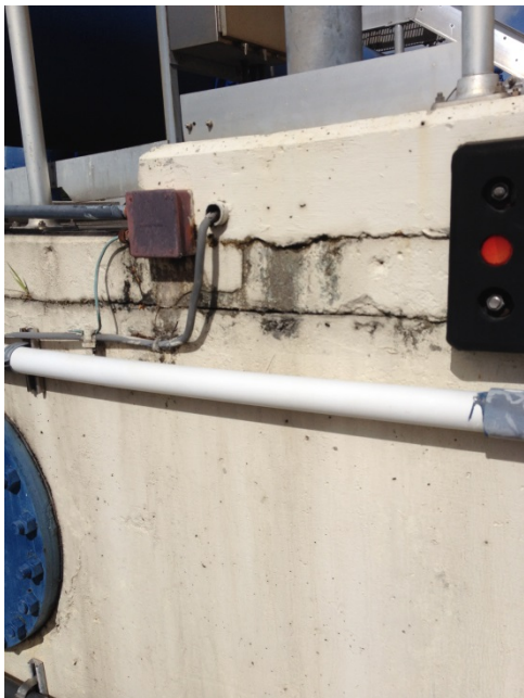
Replace expansion joint
