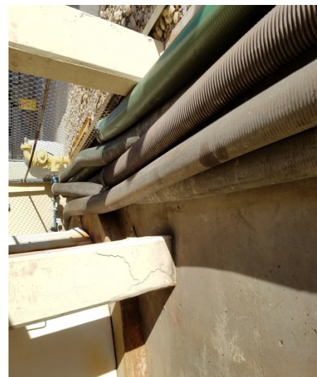
Repair cracked pillar
