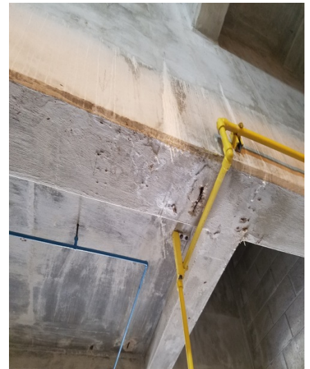
Deteriorated Ceiling Beams
