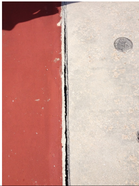
Replace expansion joint
