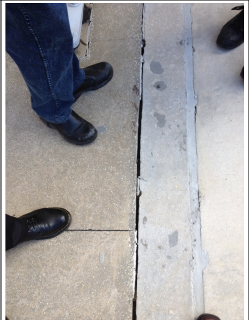
Replace expansion joint
