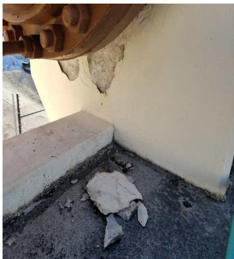
Repair Pipe Supports
