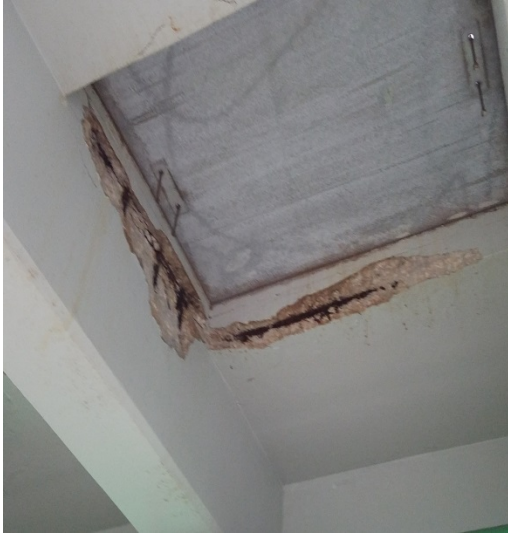
Spalling to Rebar Around Hatch
