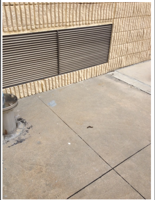
Replace expansion joint between fluted block wall and concrete slab.
