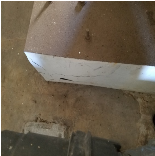
Repair Cracked Pedestal
