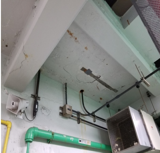
Repair Cracked Beam
