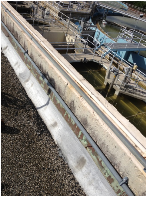
Install flashing on top of parapet
