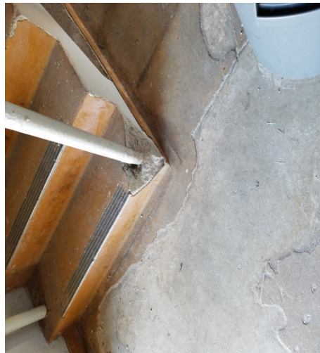
Repair Chipped Stair
