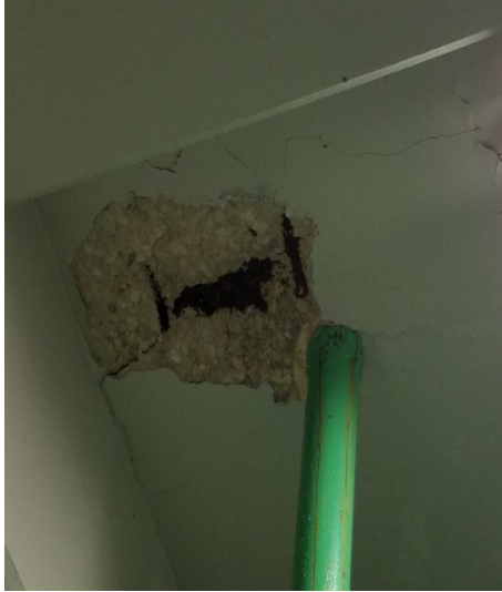
Spalling to Rebar Near Support
