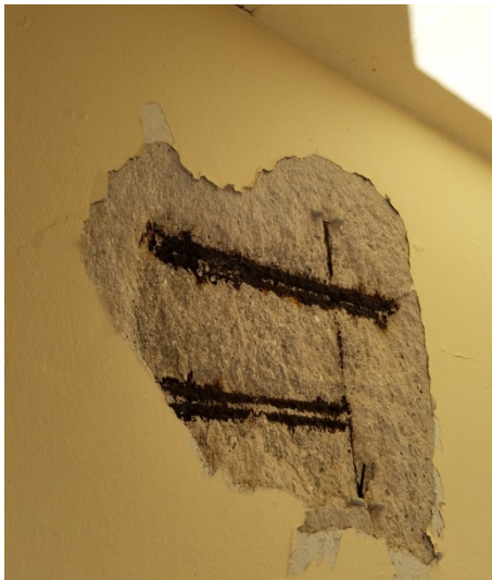
Spalling to Rebar
