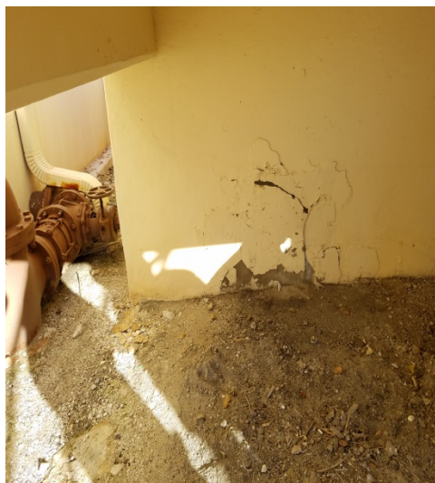
Repair Spalled Concrete
