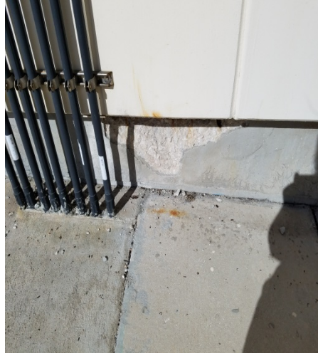
Repair Spalled Concrete
