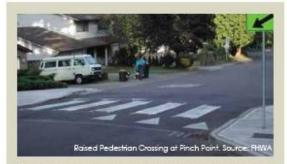
The pedestrian crossing is raised to give motorists and pedestrians a better view of the crossing area, Because of the elevation change, traffic is slowed. The raised crossing will be accompanied by a pinch point to reduce the crossing distance for pedestrians and further calm traffic.
