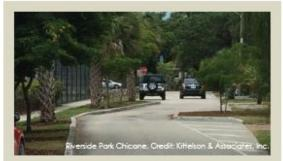
A series of fixed objects, usually extensions of the curb, which alter a straight roadway into a ziazaa path to slow vehicles. Chicanes reduce the speed of motorists but are still easy to navigate. They facilitate one- or two-way traffic. The exact design will be determined in the design phase based on further input.
