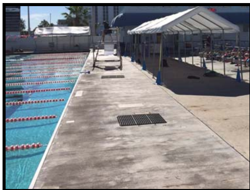
Figure 169 Access panels along pool side to drainage pipes below
