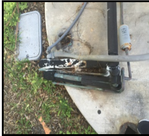
Figure 28 Refrigerant piping missing
