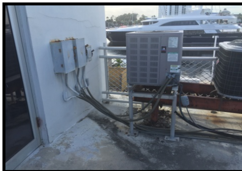
Figure 79 visible rust throughout unit
