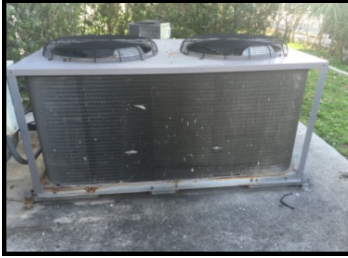
Figure 26 15 ton condensing unit, rusted
