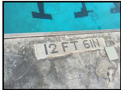
Figure 158 Light junction/transformer box in deck
