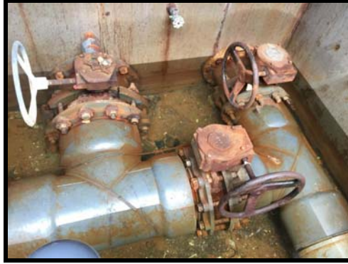
Figure 162 Standing water in vault poses safety concern, and fluctuated with the tide per FLAC staff. BECSys5 flood sensor will disable power to the circulation pumps in the event of an unsafe level of water in the tank.
