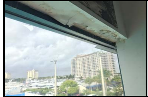
Figure 8 Building 1, second floor interior looking west. Water intrusion around window and possible mold underneath.
