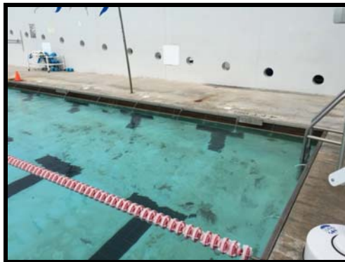
Figure 153 Interior pool plaster, the pool has never been resurfaced since it was built in 1992
