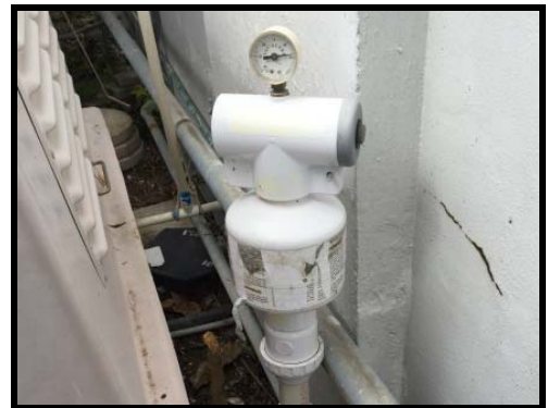
Figure 189 Some of the units have been retrofitted to comply with recent Federal Guidelines such as the direct suction line which now includes the use of a “Vac-Alert” anti-entrapment device
