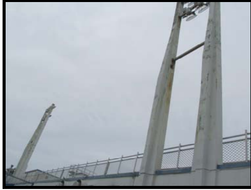
Figure 40 Exterior event lighting, showing rust stains and peeling paint
