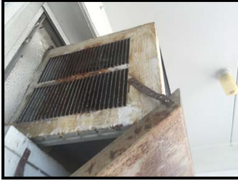
Figure 44 rusted wall air conditioning units
