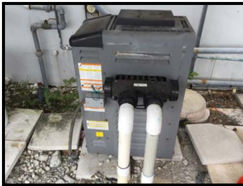
Figure 188 The existing gas heater is in fairly good condition. It can continue in operation regular maintenance by FLAC Staff
