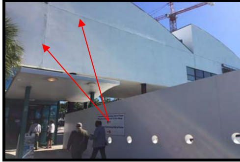
Figure 7 Building 1, west elevation, buckling at the seams in the stucco
