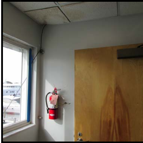
Figure 63 Building 3 window, top of stairs, water intrusion at window, ceiling and wall behind fire extinguisher
