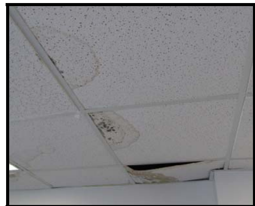
Figure 66 Building 4, meeting room ceiling on first floor, water damage and mold
