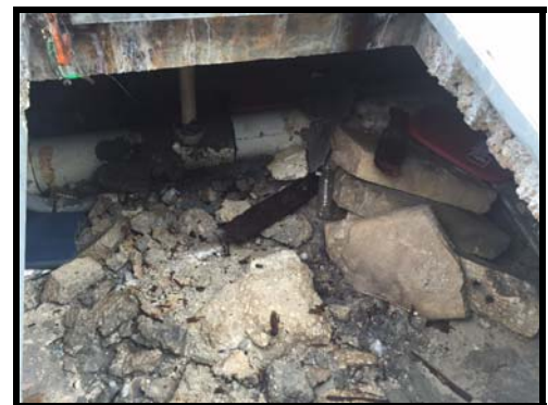
Figure 170 Underground access view of drain pipes that run parallel to pool
