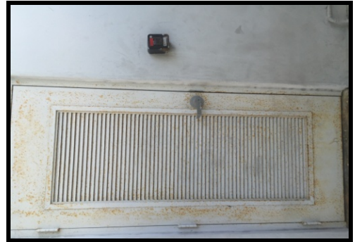
Figure 20 Damaged (rusted) door
