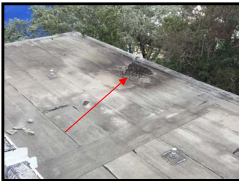
Figure 122 Roof over library, dark spot indicates pooling water damaging the roof membrane
