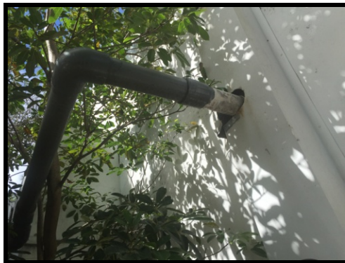
Figure 142 condenser water pipe through building needs sealant/caulk
