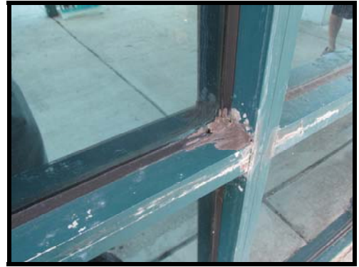
Figure 12 Exterior gift shop, patched corner of rusted storefront window frame
