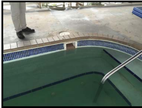
Figure 184 Skimmer section grate cover and handrail anchor, non-compliant, but allowed
