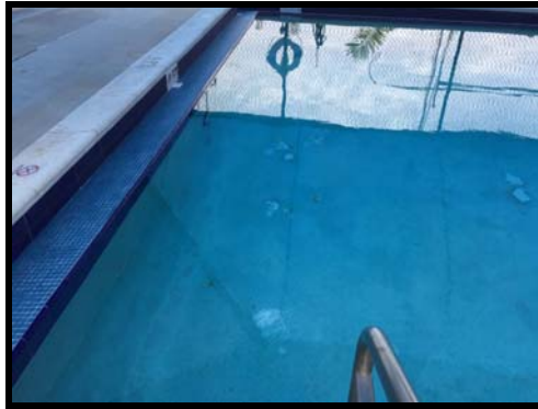
Figure 191 Interior finish is rough and stained
