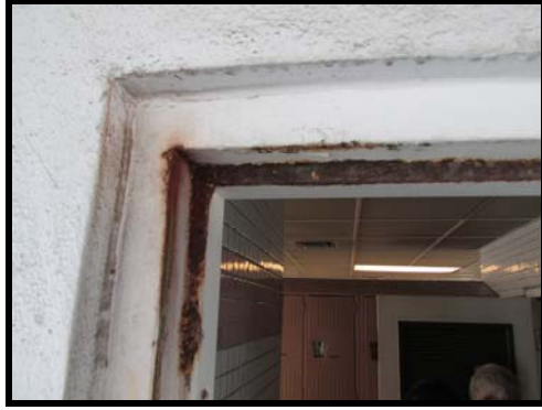
Figure 59 Exterior door on west side of Building 3 going into women's locker room, showing rusted door frame
