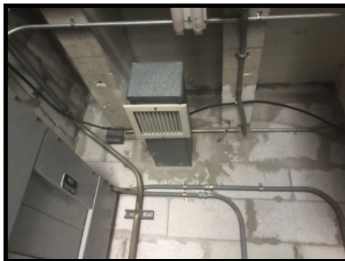
Figure 75 electrical room, exhaust inoperable
