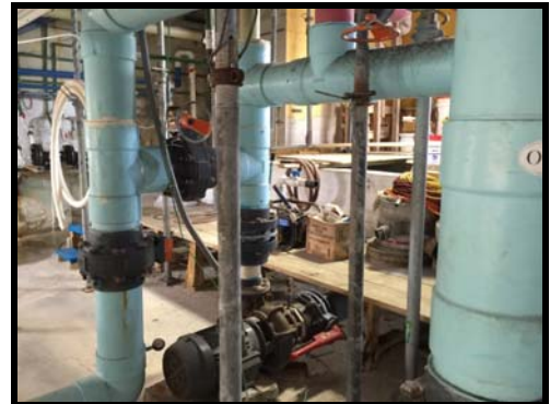
Figure 174 The pool equipment "face piping" is in excellent condition and there are no signs of leaking pipes in the room
