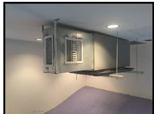
Figure 18 mechanical unit in Proshop stair up to second floor, not easily accessible
