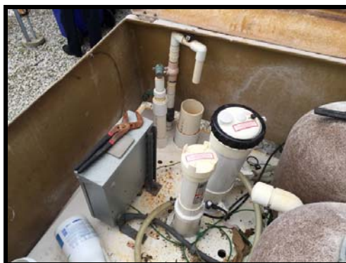
Figure 186 Manual pH feed, lack of chemistry control, and use of Bromine are a major cause for concern in a small body of water.
