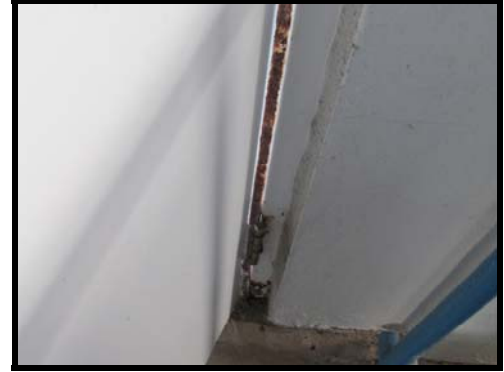
Figure 60 Exterior door on west side of Building 3 going into women's locker room, showing rusted door frame
