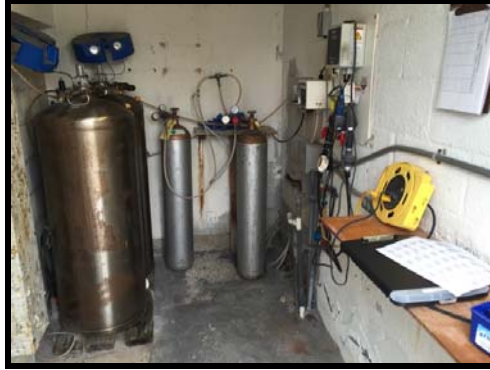
Figure 161 Co2 system, circa 1994 requires repair or replacement, and its inefficient use of Co2 gas is costing the City additional money every month
