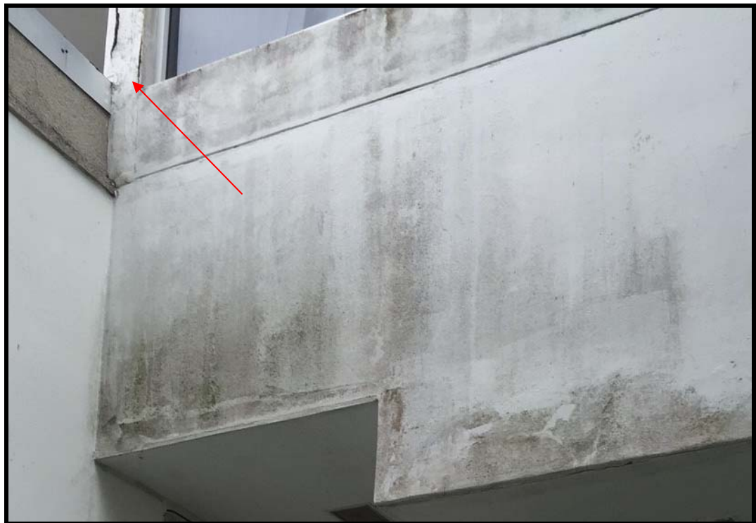
Figure 117 Exterior of Building 5 at northwest exit stair, showing cracked and deteriorating stucco allowing water intrusion
