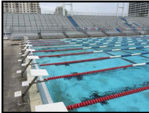
Figure 171 Starting blocks are old and broken in various degrees, such as platforms, grips, and Anchors. The blocks are vastly outdated and lag far behind current models in use at other facilities
