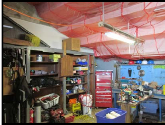
Figure 38 Interior maintenance/storage area, safety netting installed to prevent concrete falling on occupants. Hard hat area.
