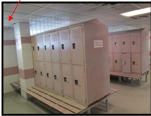
Figure 67 Building 3 women's locker room, showing uneven grid
