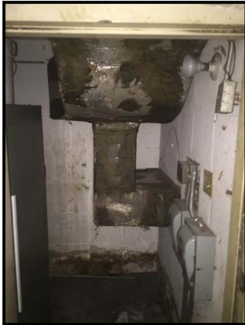
Figure 130 low ductwork in mechanical space above restrooms in banquet area
