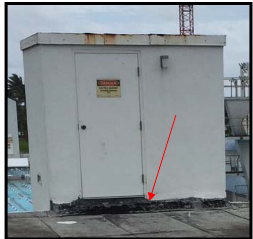
Figure 127 Deteriorating roofing material at elevator tower causing leaks and water damage below
