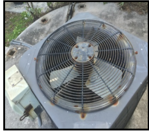
Figure 29 2-5 ton condensing unit, worn and rusting
