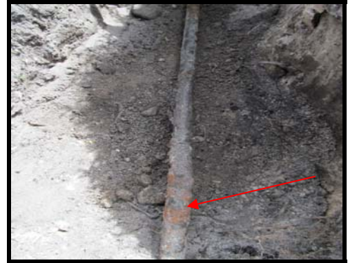
Figure 200 Tie back: exposed section of seawall tieback, condition of steel is very good, slight section of rust which was directed to be re-coated
