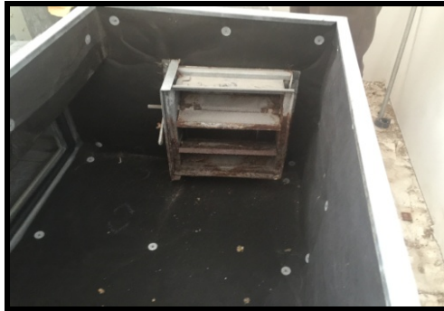
Figure 19 Outside air intake damper
