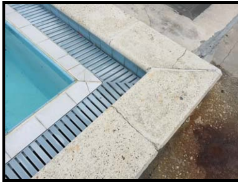
Figure 167 Gutter at perimeter of pool
