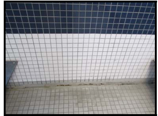
Figure 70 Building 3, men's locker room, cracked and deteriorating sealant
