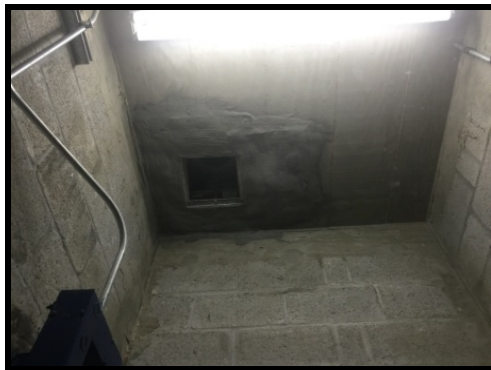
Figure 21 Non-ventilated telecom closet
