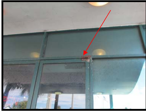
Figure 11 Building 1, exterior storefront door entering gift shop, rusted door hardware
