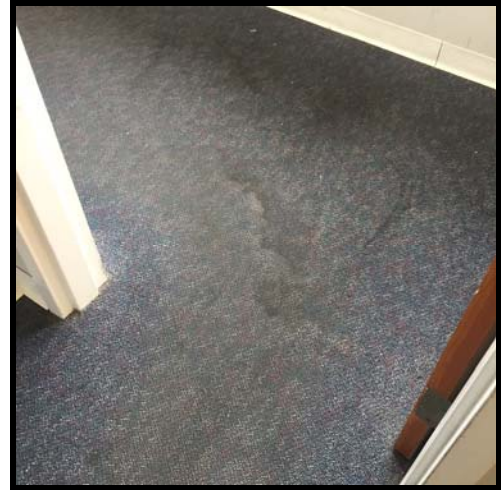
Figure 64 Building 3, top of stairs, water damage from window and roof
