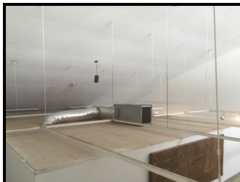
Figure 17 mechanical unit above ceiling space
