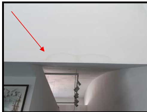
Figure 9 Building 1, water stain on interior intersection of curved roof.
