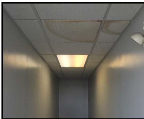
Figure 65 Ceiling above stairs in Building 3 showing water damage
