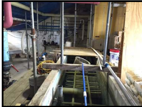
Figure 173 DE system is functional and could be utilized in Option 1, but is very labor intensive and created additional demands for storage, use, and disposal of potentially carcinogenic DE powder
