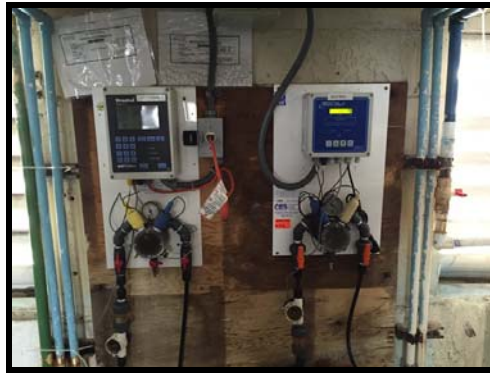
Figure 175 Competition pool and Dive Well controllers, CES circa 1990's are in need of repair or replacement
