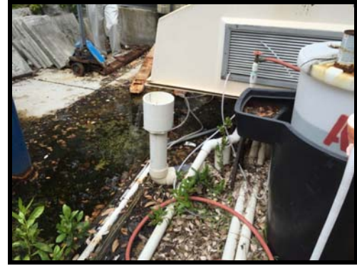
Figure 194 Equipment Vault Piping and other components have been retrofitted to relate top site conditions. The pool drain line is no longer connected to the Atmospheric Gap Funnel Drain and is routed to site drainage elsewhere beyond the perimeter wall.
