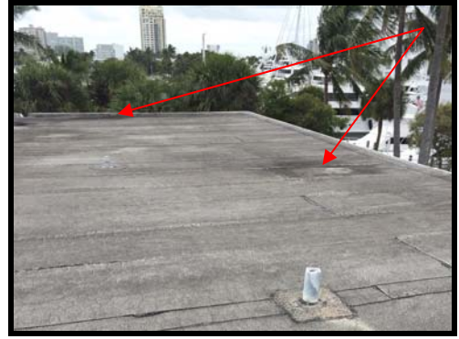
Figure 121 Roof over main exhibit space, dark spots indicate standing water causing the membrane to detach and bubble
