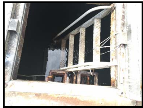
Figure 181 Ladder into dive observation room, corroded and filled with water
