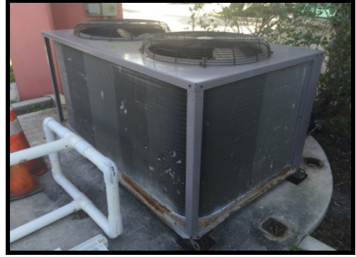
Figure 27 10-15 ton condensing unit, rusted
