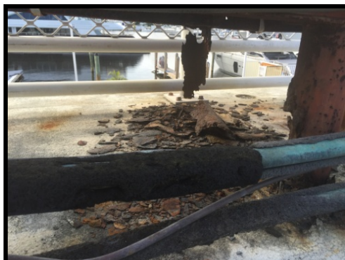
Figure 81 serious deterioration of the coil fins
