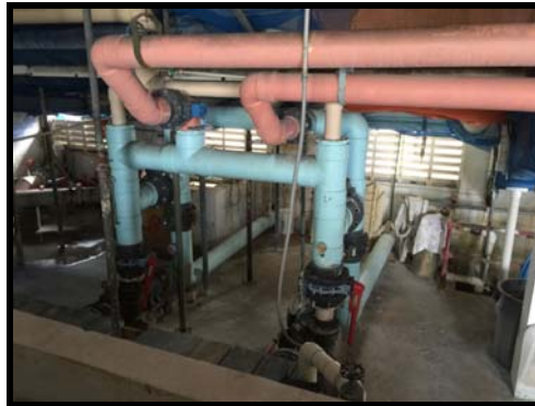
Figure 177 The pool pumps (2) and vacuum D.E filter system is currently operational and performing well. The geothermal heat pump units are also in good condition and performing well. The room lighting is inadequate. It is required by code to have 30 Fc of illumination at the floor level
