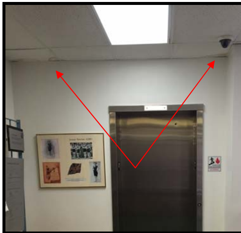
Figure 126 Second floor elevator lobby indicating water damage to ceiling tiles from roof above
