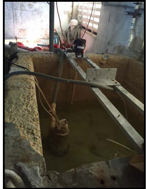
Figure 37 Interior pump room, chemicals deteriorating concrete
