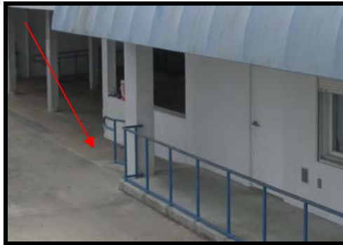
Figure 53 Ramp on north side of Building 4, ramp not long enough, slope too steep
