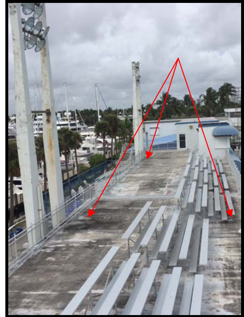
Figure 58 Observation deck between Buildings 3 & 4, showing dark spots indicating pooling of water and water damage
