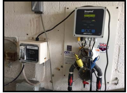
Figure 160 Circa 1994 controller is in need of repair or replacement, and does not provide the control features required in a 50-meter pool facility
