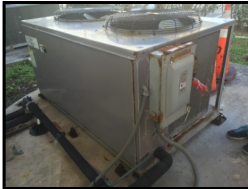
Figure 24 condensing unit
