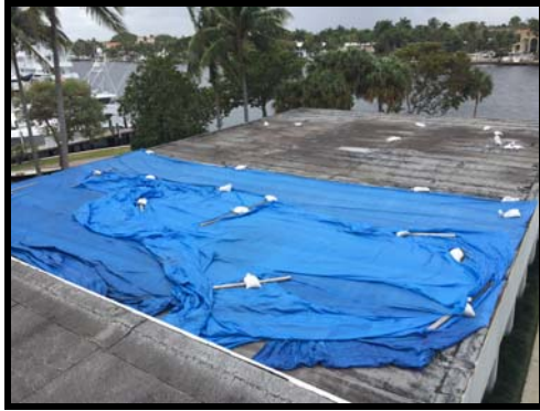
Figure 120 Roof top of banquet hall, damaged, causing major leakage on the interior
