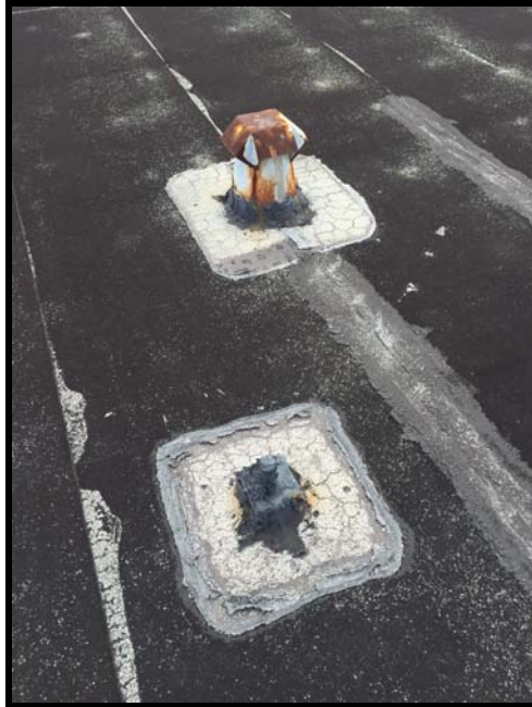
Figure 57 Roof of Building 3, showing cracked sealant around penetrations as well as between roof membrane pieces
