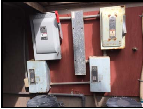
Figure 159 Starters in enclosed space can be located above grade and connected to the BECSys5/7L for direct control of pool circulation and proof of DOH flow compliance
