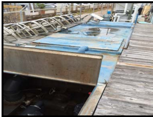
Figure 164 Paddock Vacuum Sand Filter and Pump Vault is submerged and subjected to sea water
