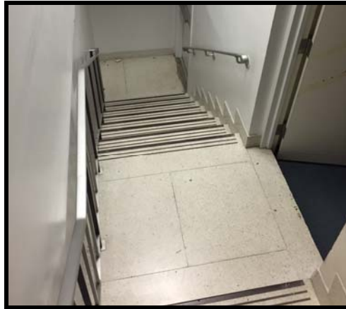
Figure 128 Stairs from office and mechanical room to outside. Railings do not comply with Florida Building Code
