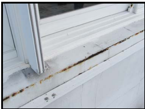
Figure 61 Window on Building 3 showing rust, peeling paint and cracks in the wall below
