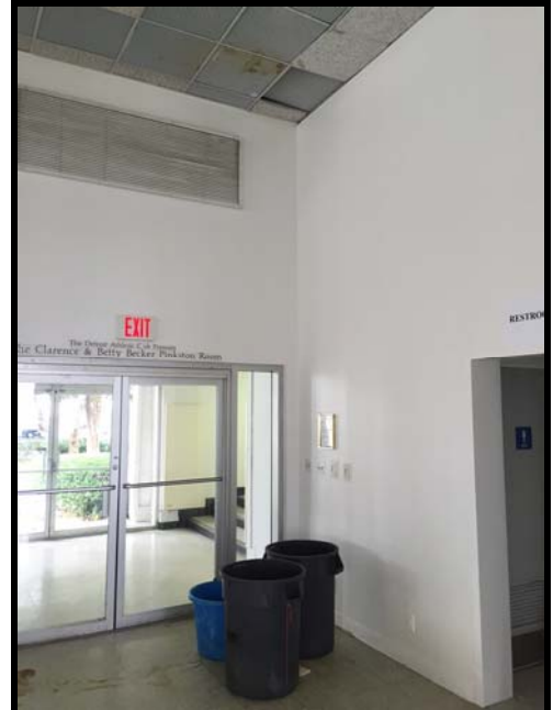
Figure 119 Northeast corner of banquet hall showing major roof leaks leading to the closing of the space to the public
