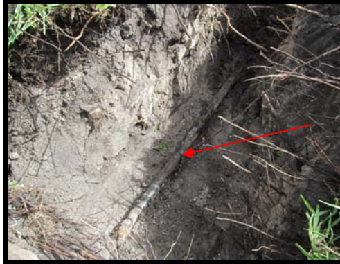
Figure 199 Tie back: exposed section of seawall tieback, condition of steel is very good
