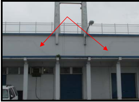
Figure 36 Exterior showing cracks in stucco
