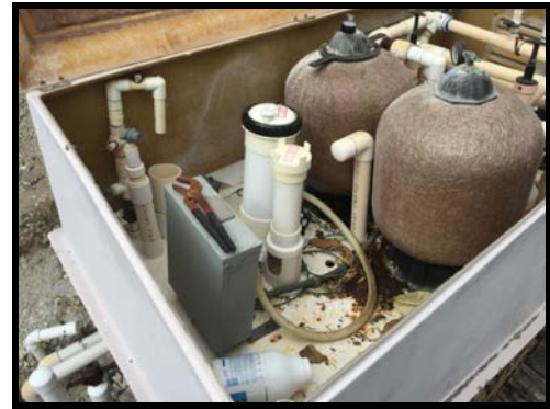
Figure 185 Diver Warmup Spa is in disrepair and can be replaced by either a pre-plumbed pack, or the components can be site assembled and a prepared slab
