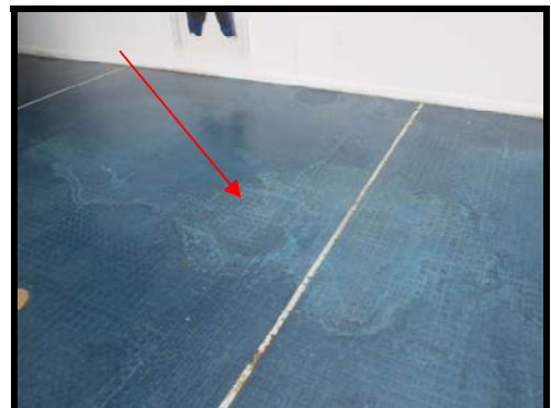
Figure 10 Previous leaks from the roof and walls causing water damage on the floor finish
