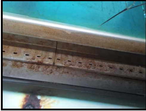
Figure 155 Stainless steel gutter, view taken from the deck above shows inside of the gutter rusting and corroding at joints and anchor points
