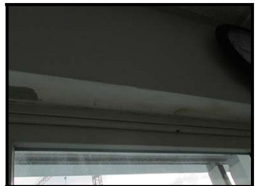
Figure 62 Window on second floor of Building 3 at top of stairs, showing water damage
