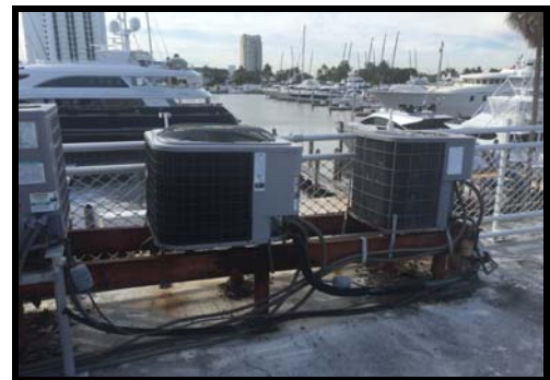
Figure 80 unit stand in poor condition
