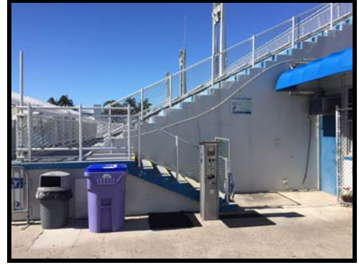
Figure 41 Exterior access to bleachers, showing inadequate railings and no ADA access.
