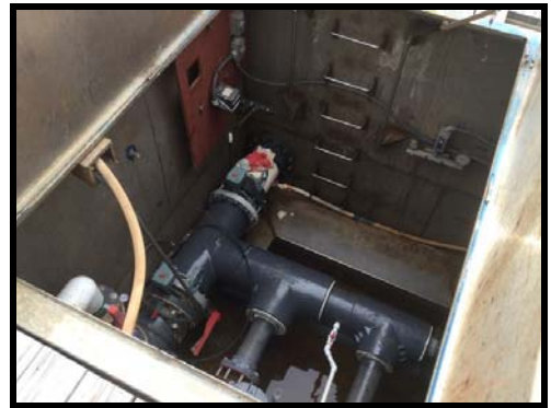
Figure 165 Training pool filtration system vault, Circa 1990 is functional but has some code compliance, safety and operational issues that need to be addressed
