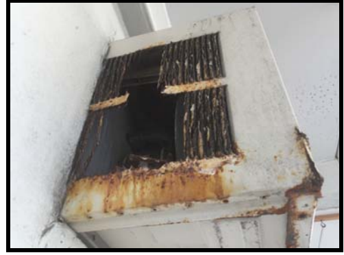
Figure 45 rusted wall air conditioning units
