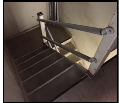
Figure 129 Stairs from mechanical room next to banquet hall. Stairs do not comply with Florida Building Code
