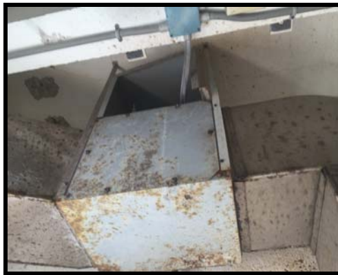
Figure 42 rusted ductwork
