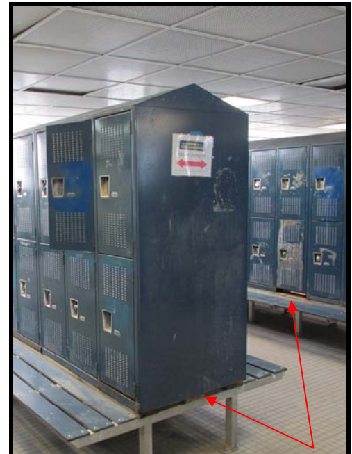
Figure 72 Building 3, men's locker room, rust along the bottom and work locker doors, sides and benches
