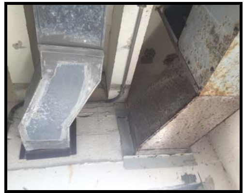
Figure 43 rusted ductwork
