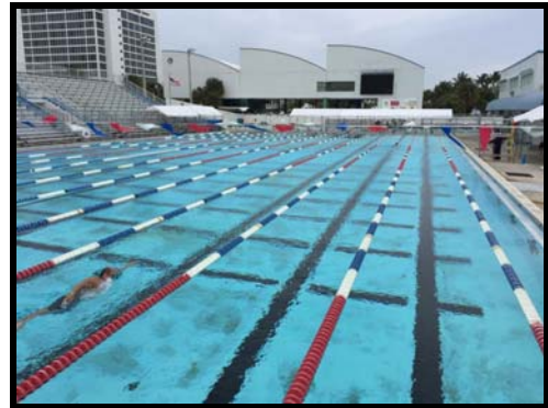
Figure 172 7'-0" wide lane width does not meet national standard lane width of 8'-2"
