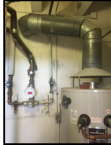
Figure 86 boiler room flue, missing sealant and water proofing
