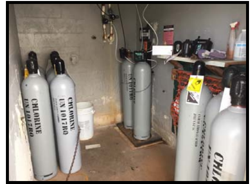
Figure 176 Gas Chlorination system is very dangerous to operators and patrons alike and should be either replaced or outfitted with scrubbers, etc. Staff certification for gas is minimal and should be revisited ASAP.
