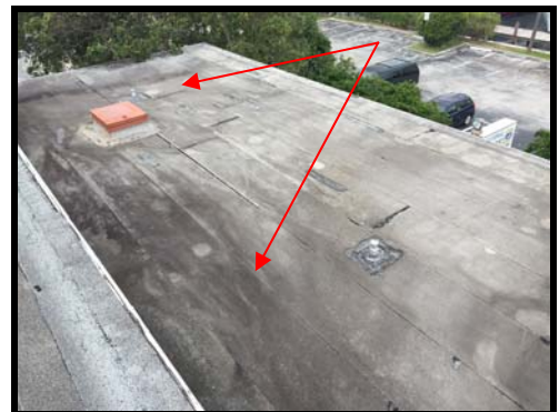
Figure 123 Roof over lobby area, showing the standing water patterns
