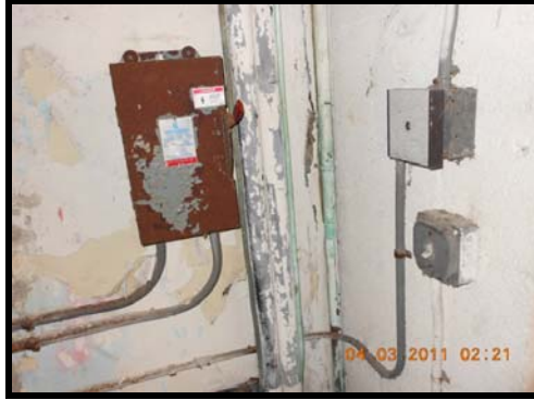
Figure 102 disconnect switch and junction box
