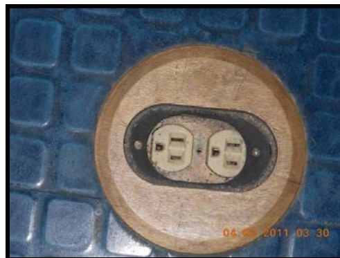
Figure 30 uncovered floor outlet
