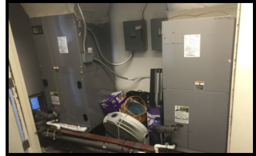
Figure 78 air handling unit
