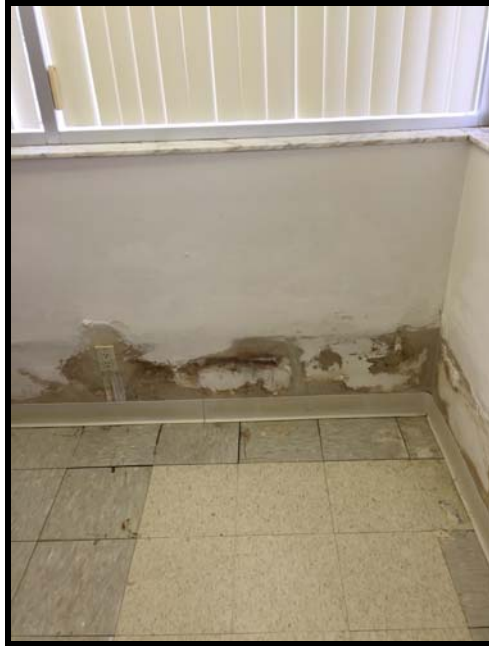
Figure 118 Second floor lunch room, southwest corner, showing severe water damage to wall and floor, rot and mold
