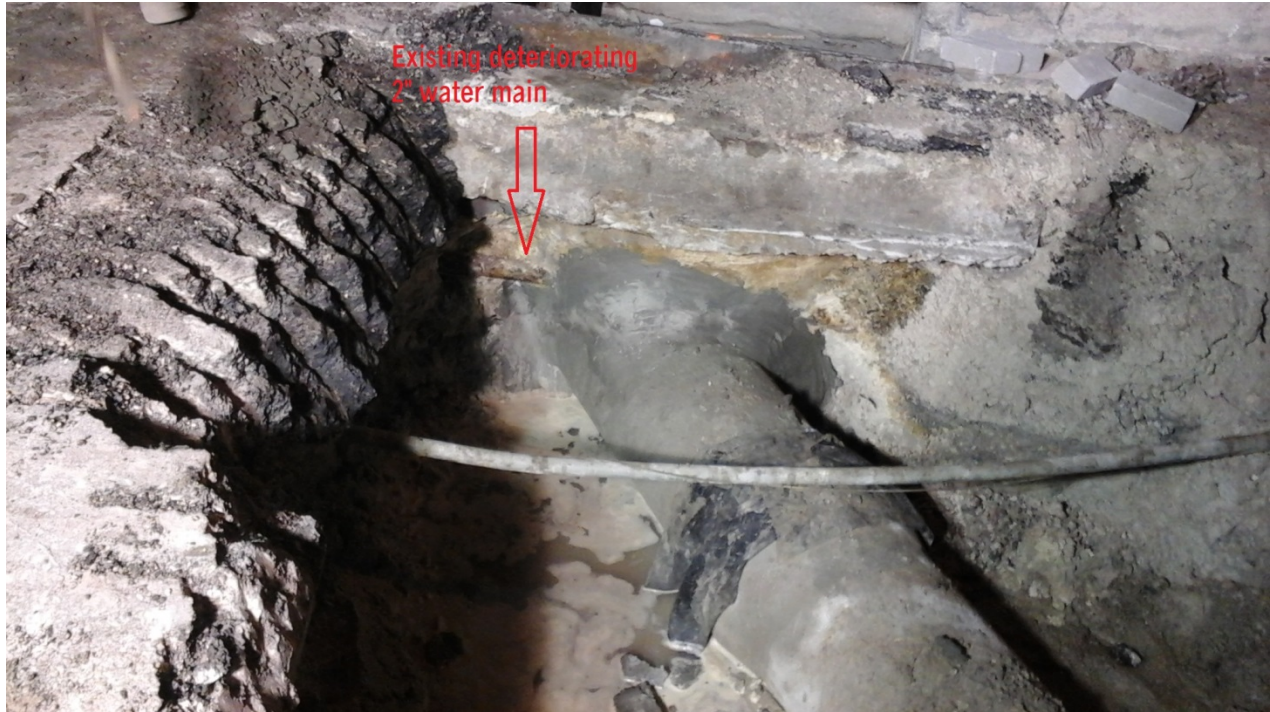
Existing Deteriorating 2" Water Main in Sunrise Boulevard – Exposed During Florida Department of Transportation's US-1 Project
