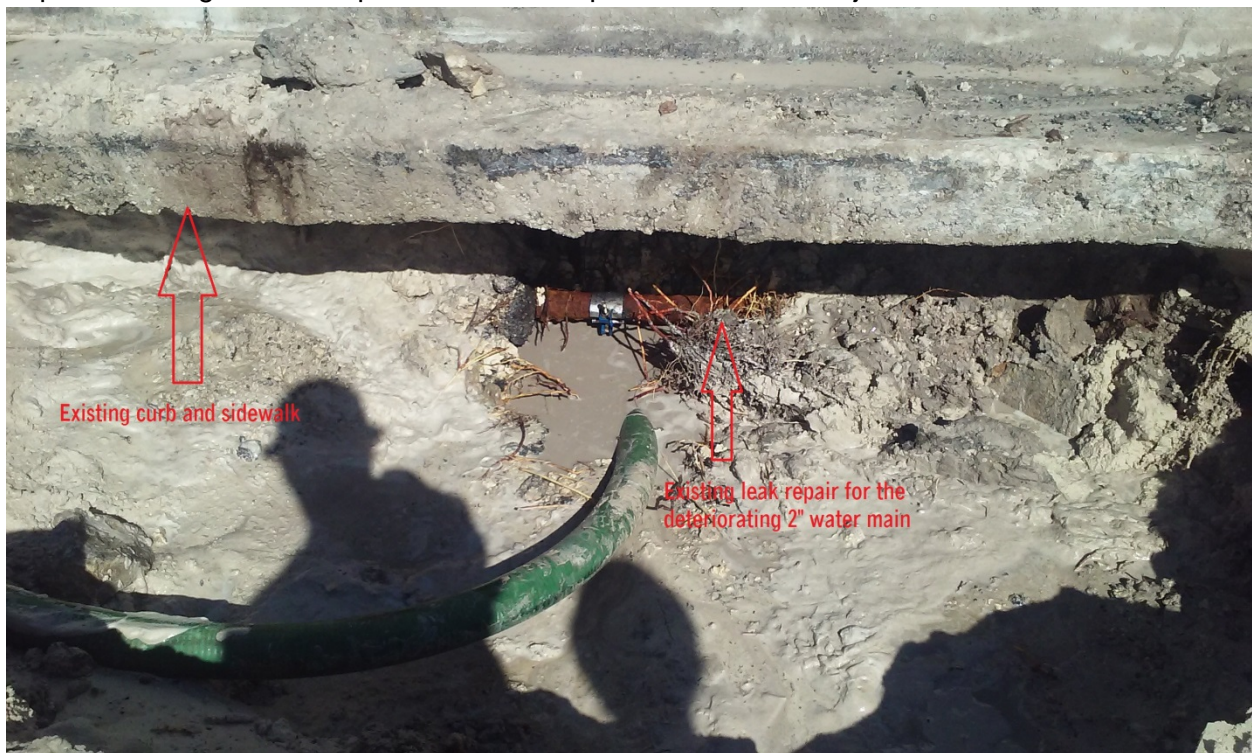
Existing Deteriorating 2" Water Main in Sunrise Boulevard – Exposed During Florida Department of Transportation's US-1 Project
