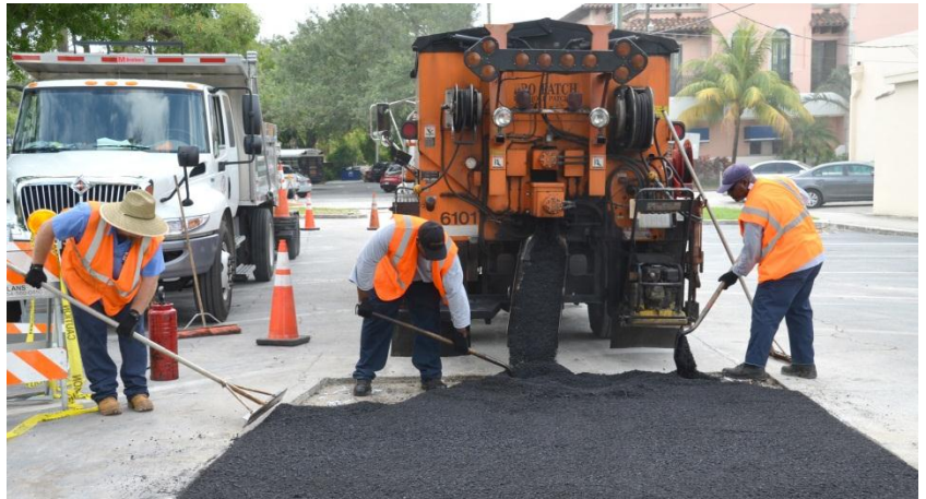
Public Works crew completing hot-in-place asphalt patching
