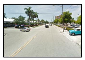
The existing conditions along Cordova Road consist of a 4-lane section within a 70 foot right of way. The roadway has sidewalks on both sides with a landscape buffer in a portion. The existing 46-feet width of paved asphalt is not pedestrian or bicycle friendly.
