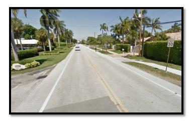
The existing conditions along Bayview Drive consist of a 2-lane section within a primarily 80 foot right of way. The roadway has a 3 foot shoulder, and sidewalks on one side with a landscape buffer. The existing 29-feet width of paved asphalt is not pedestrian or bicycle friendly.
