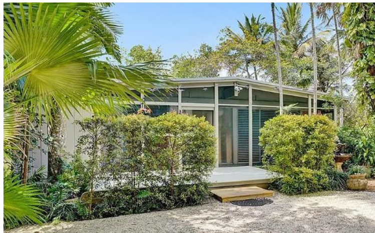
Existing Single-Family Residential Structure
