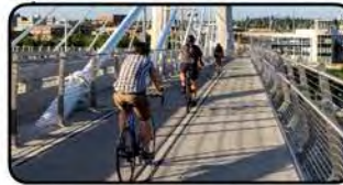
Bridge Multi-Use Paths
