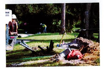
directional boring or horizontal directional drilling, installs underground piping to safely place our electric cable to connect power to your home or business. Unlike open trenching, directional boring allows FPL to install underground equipment while minimizing impact to trees and other vegetation on your property. The underground facilities will be installed 36 inches to 48 inches below the surface, or deeper, if necessary, to avoid tree roots.
