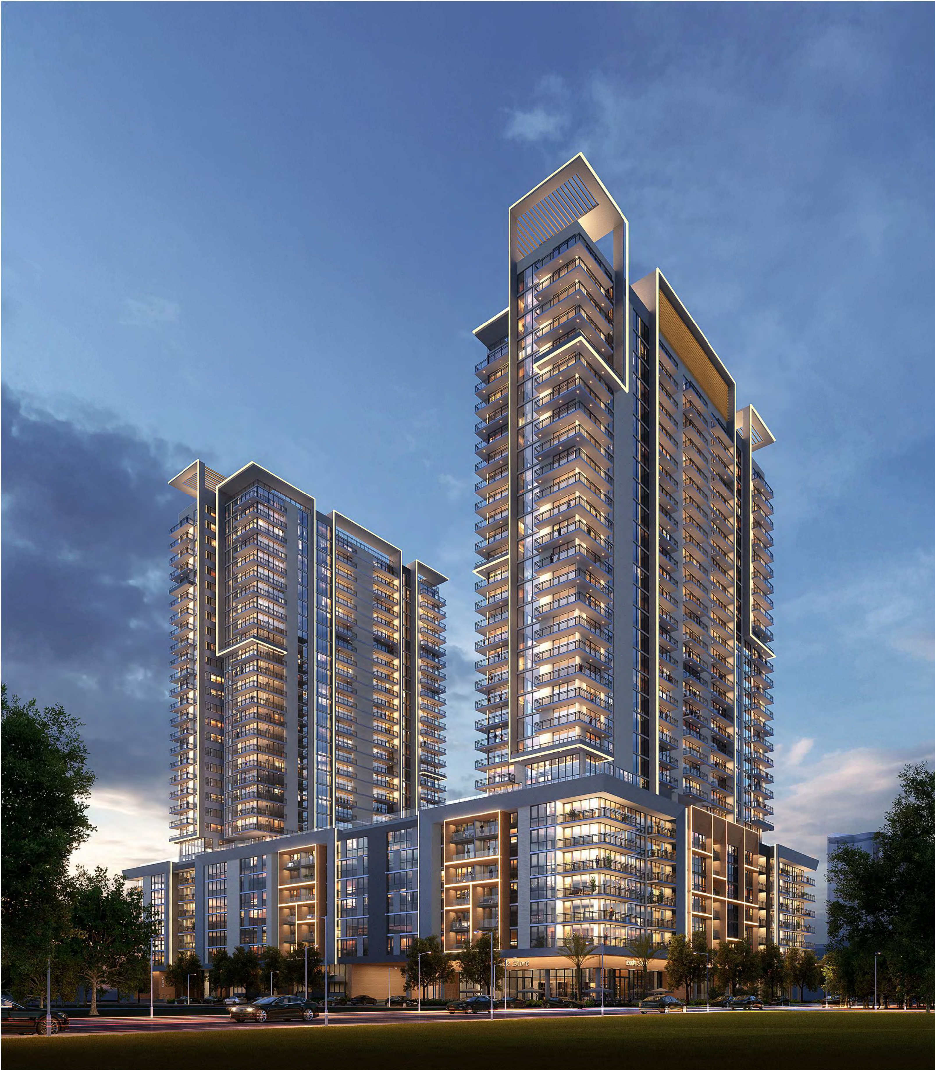
SE CORNER - ELEVATED VIEW
