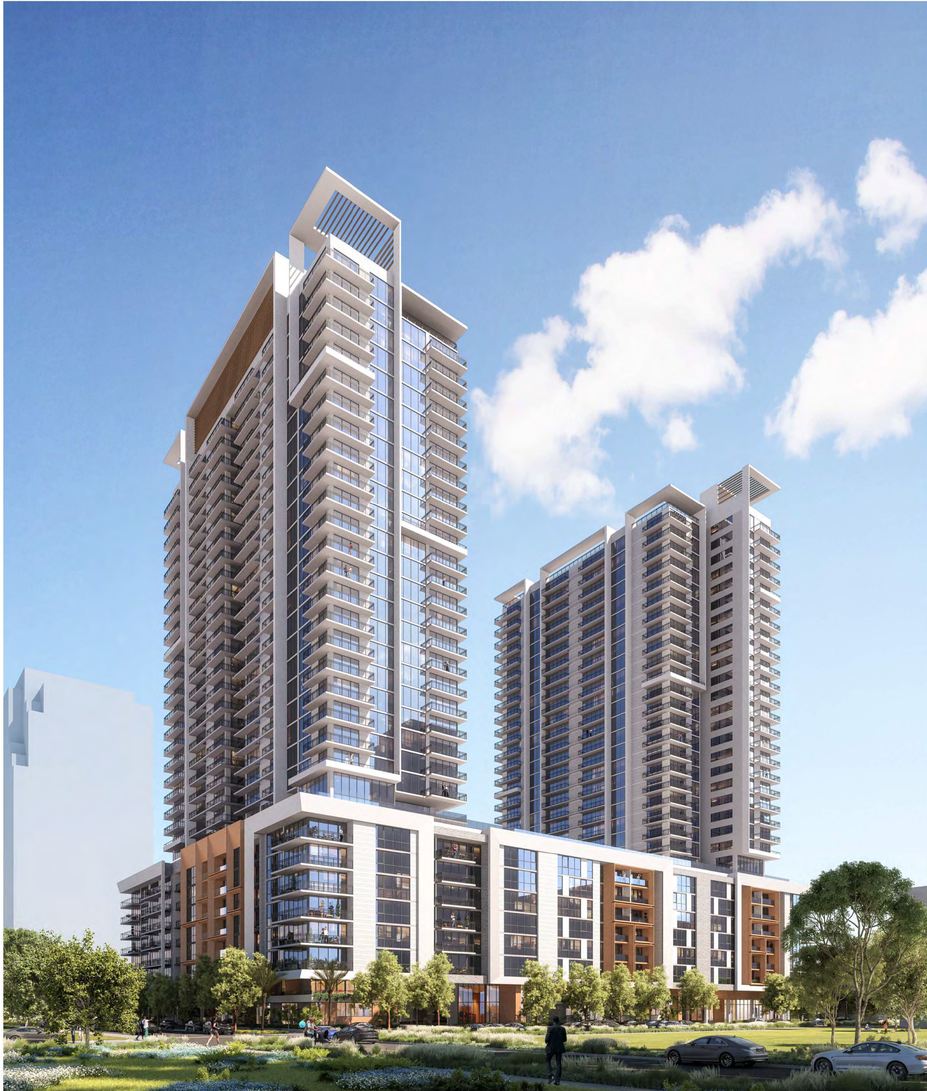
SW CORNER - ELEVATED VIEW
