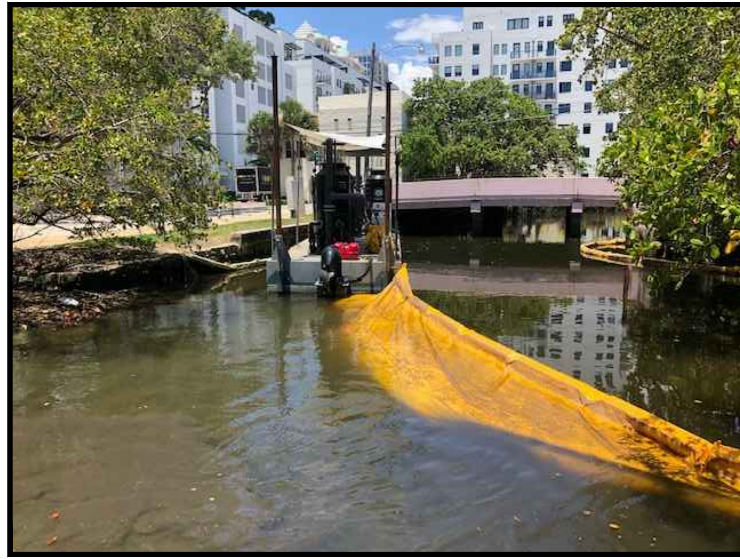
PHOTO 3: TURBIDITY BARRIER AND BARGE AT NORTHWEST END OF HIMMARSHEE CANAL. (WEST VIEW)
