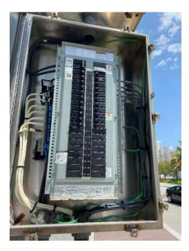
The larger service points can be described as load centers. Load centers are typically 240/480 volts or 120/240 volt electrical panels with the capacity to power more than three circuits. Typical load centers have one or two spare circuits and a hand-off automatic selector switch. These panels can be used to power many lights and receptacles.
