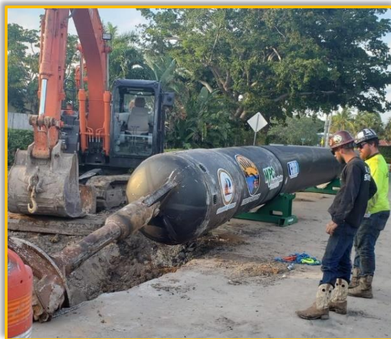
Installation of pipe through directional drilling
